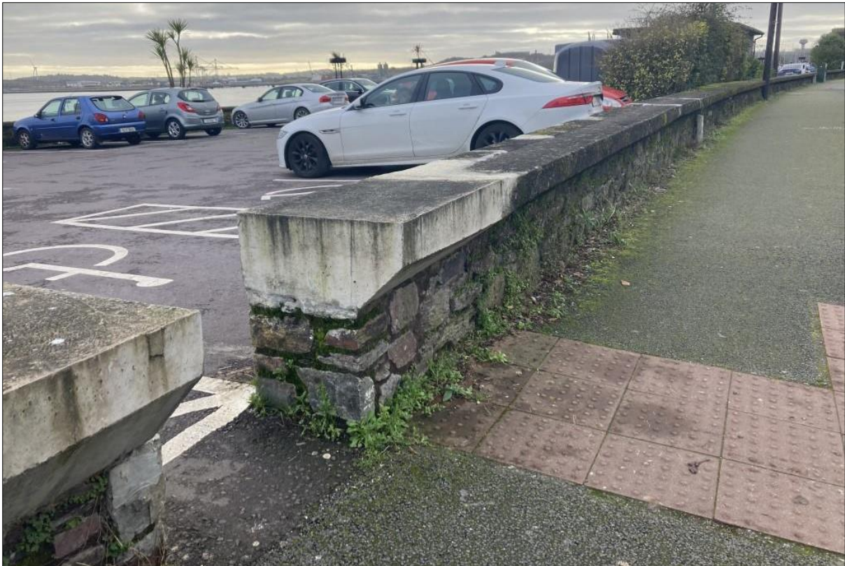
Plate 4: Modern opening in wall with replacement concrete capping
