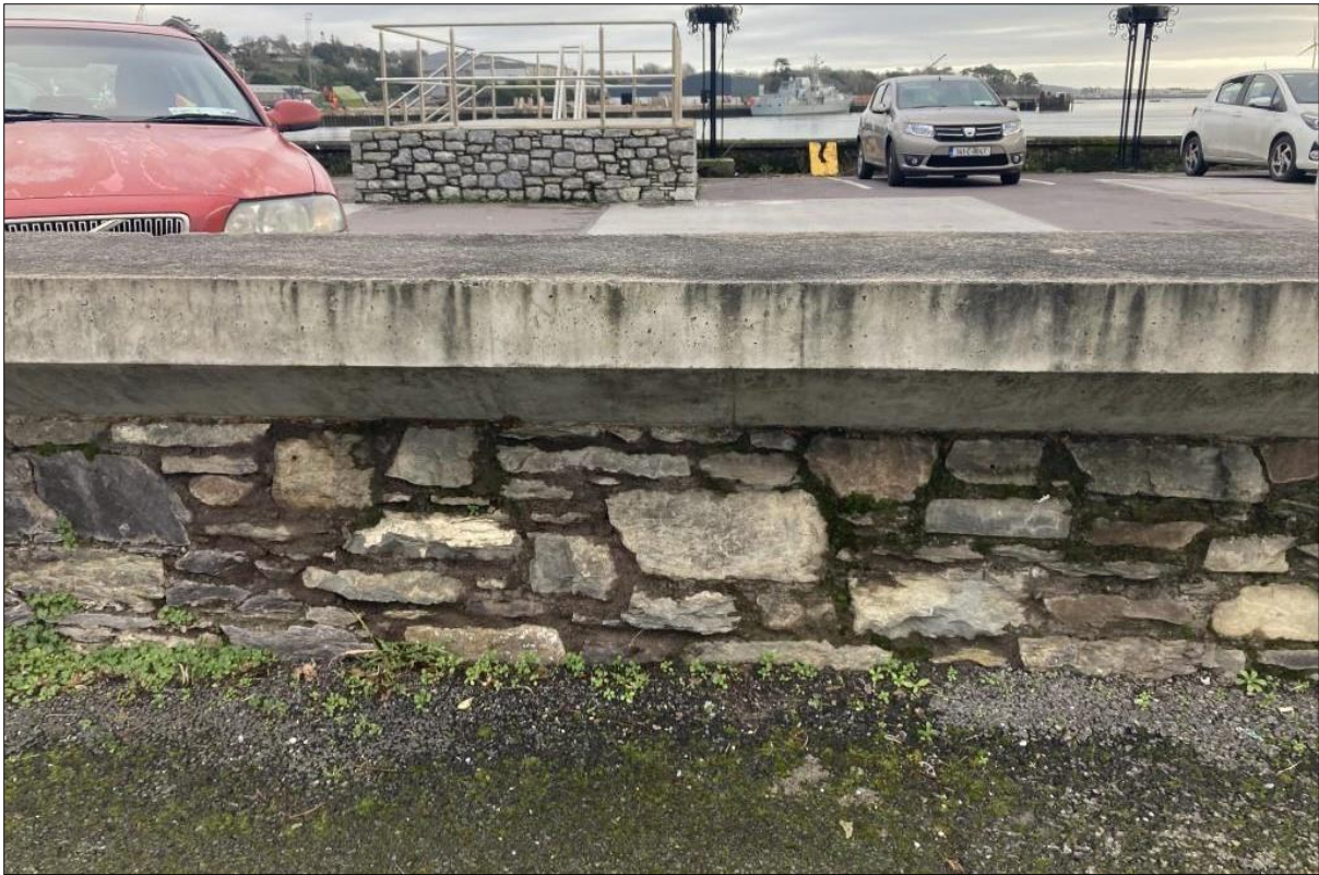
Plate 6: Rebuilt portion of wall (with modern cast concrete capping)
