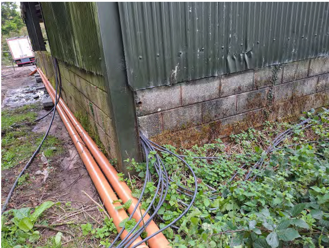
Photo 7. Electricity Supply Cables from Generator to Mobile Homes.
