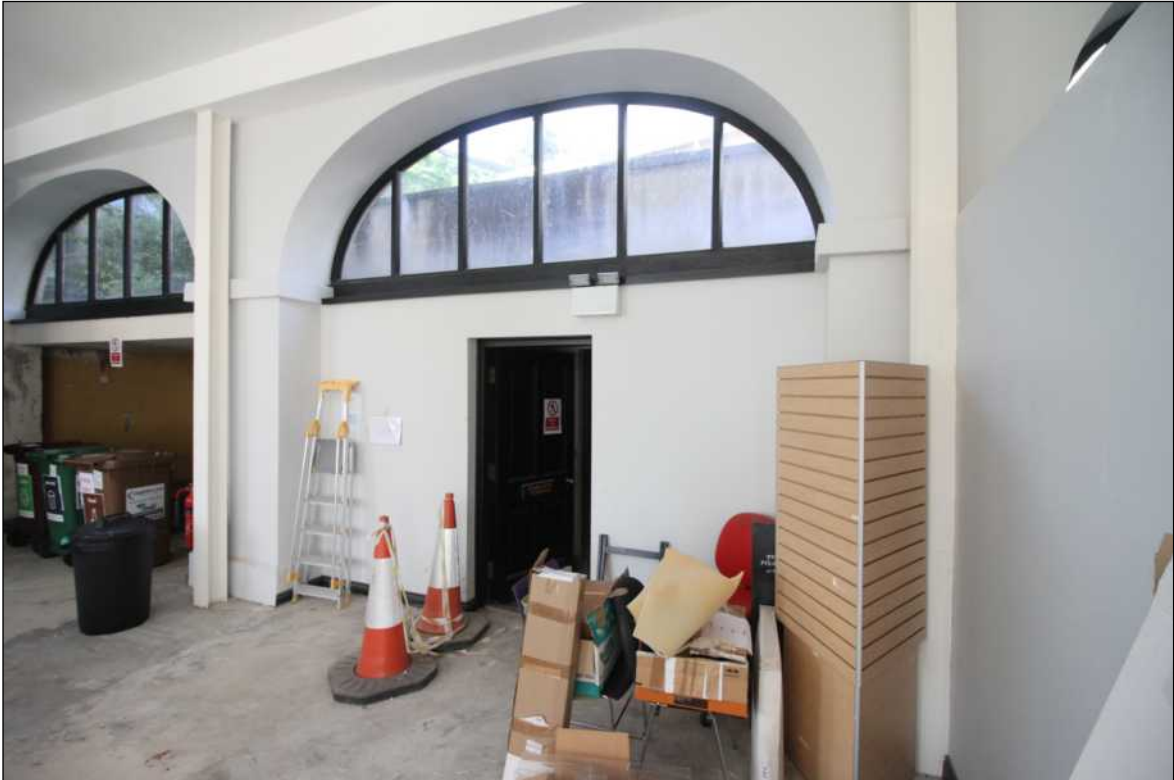
• Fig 61. Room 9. Rear flat North roofed rooms under arches.
