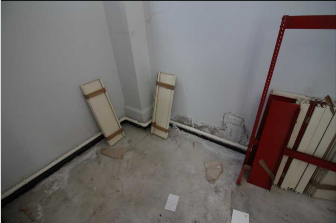
• Fig 65. Rear North Room No. 12.
