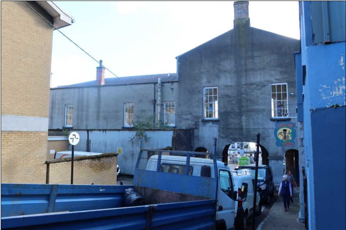
• Fig 18. North elevation and view through arch to Casement Square.
