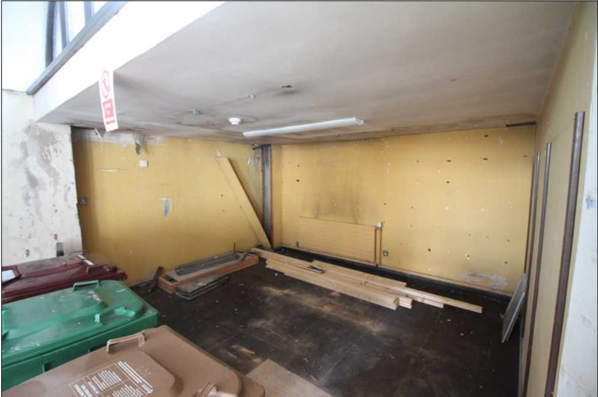
• Fig 63. Room 10. Rear flat North roofed rooms.
