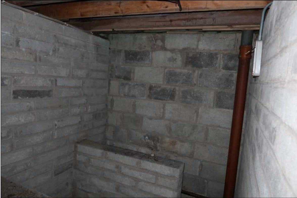
• Fig 70. Room 11. Rear North flat roofed rooms .
