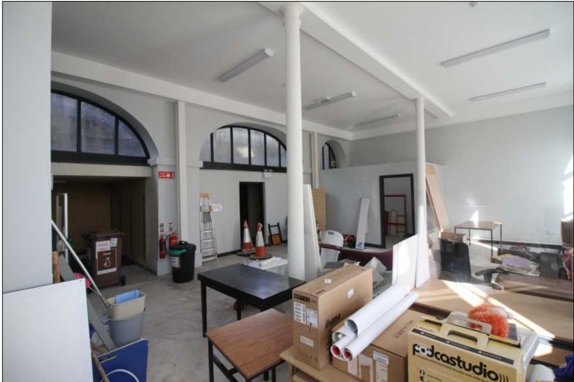
• Fig 58. Room 9. Former Childrens reference and lending, and view to NE corner.
