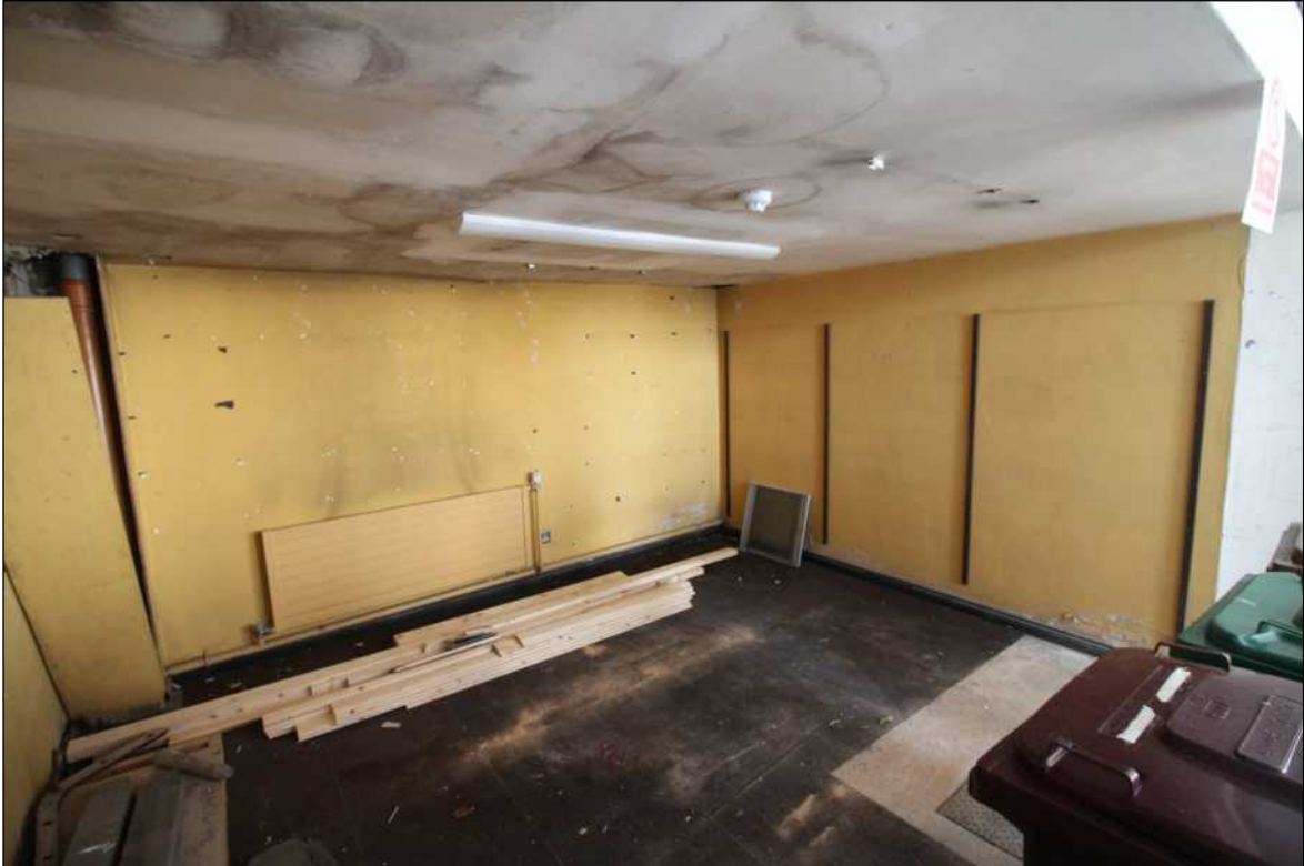
• Fig 62. Room 10. Rear flat North roofed rooms.
