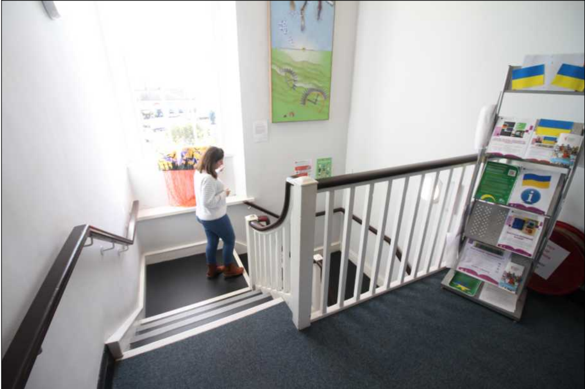
• Fig 43. Middle main access stairs. Room 8.
