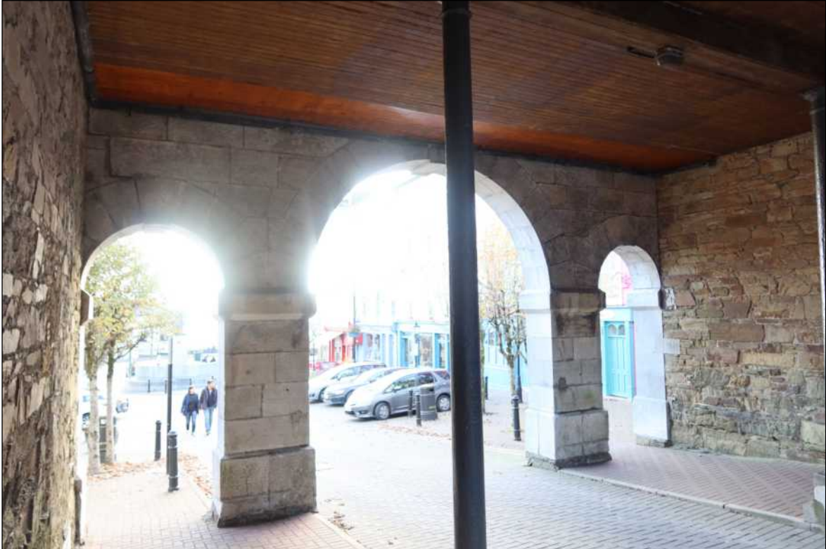
• Fig 15. Building undercroft looking South.
