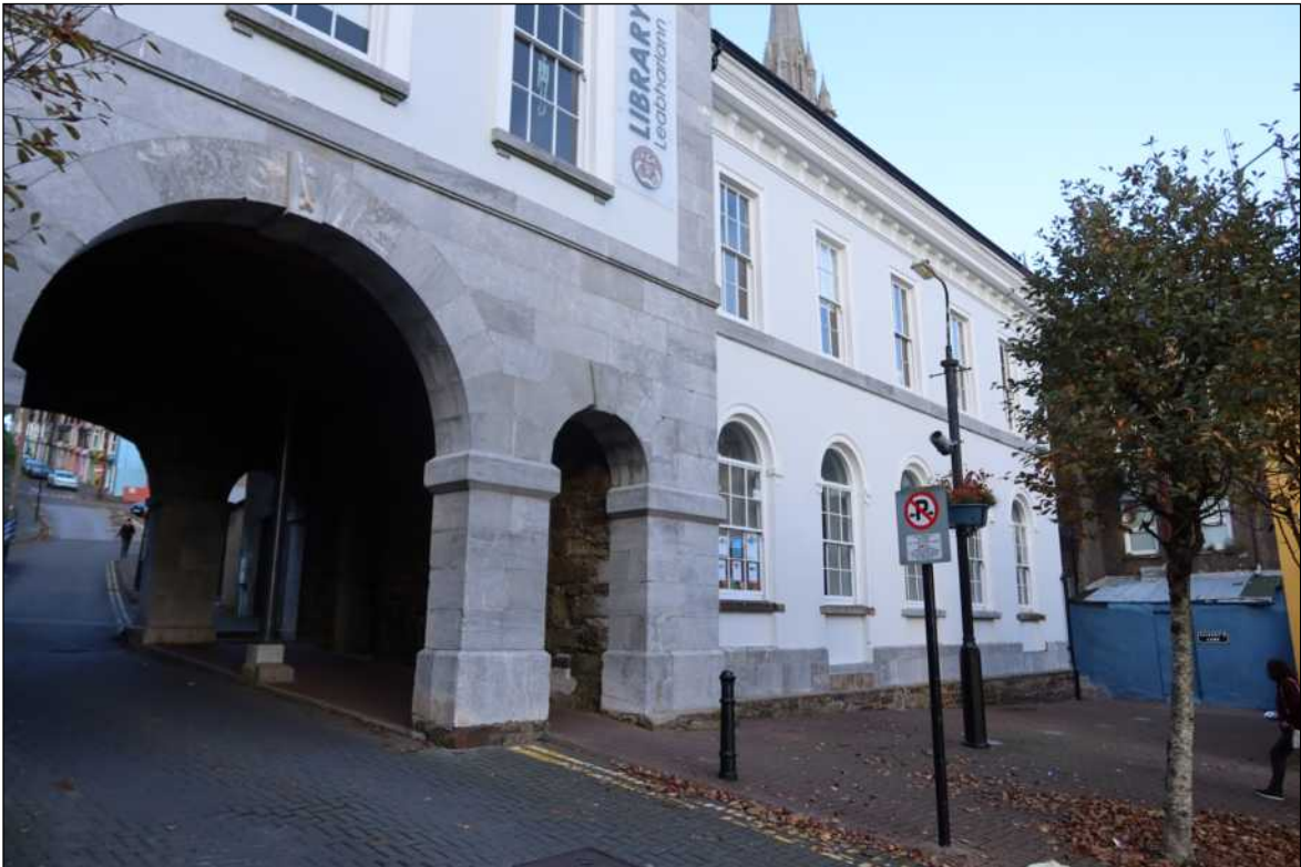
• Fig 12. South elevation and East wing, now housing library on upper level and site for new Hub below.
