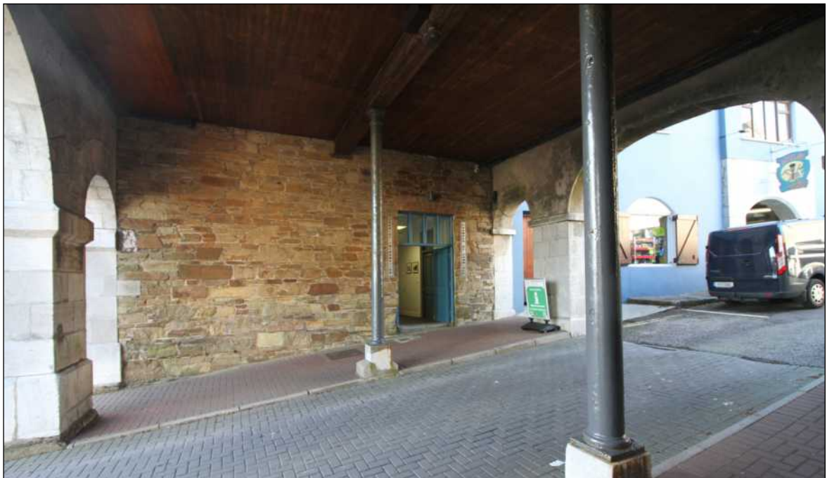
• Fig 9. Arch fronted road crossing under building.
