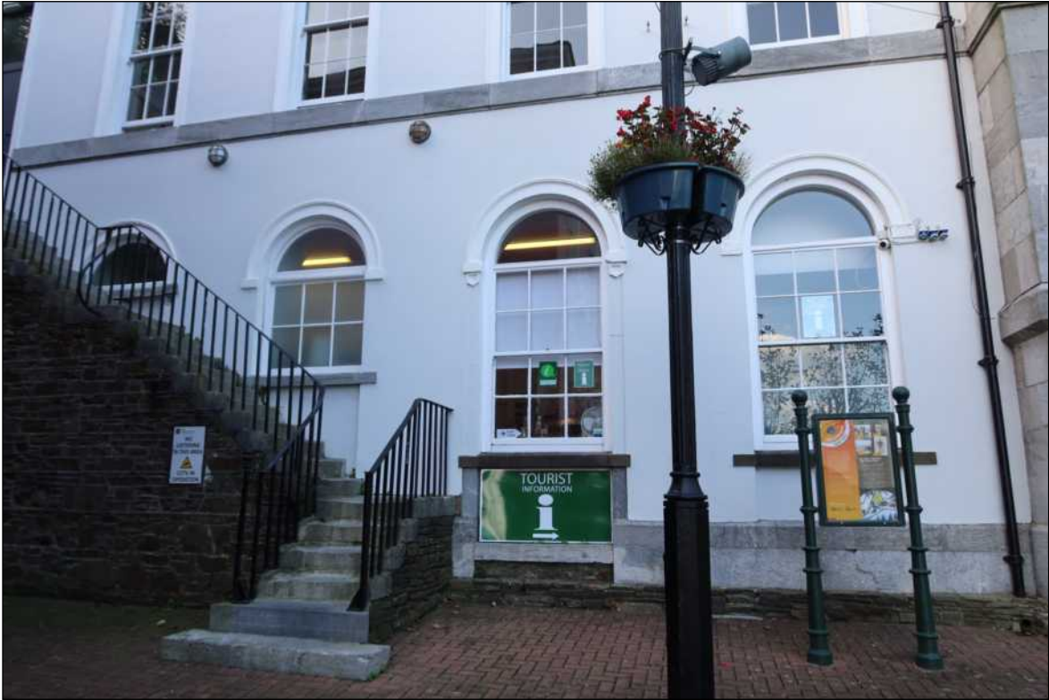
• Fig 13. West elevation with tourist office to ground floor
