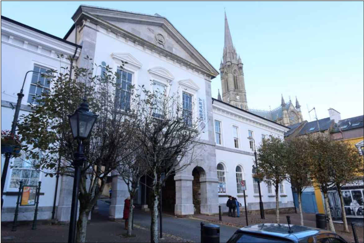
• Fig 11. South elevation and St. Finbarrs Cathedral behind.
