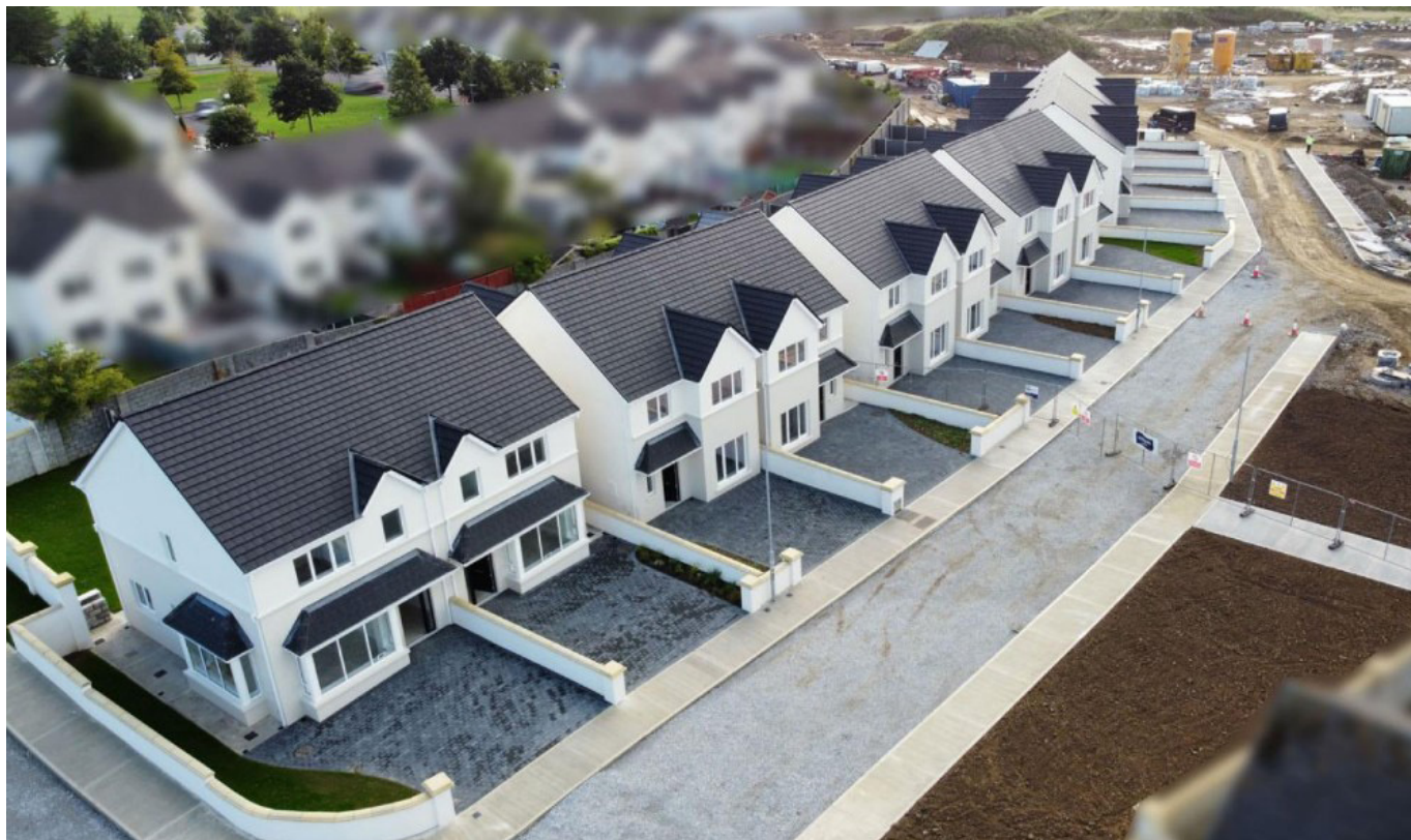
Completed Affordable houses in Clonmore, Mallow.
