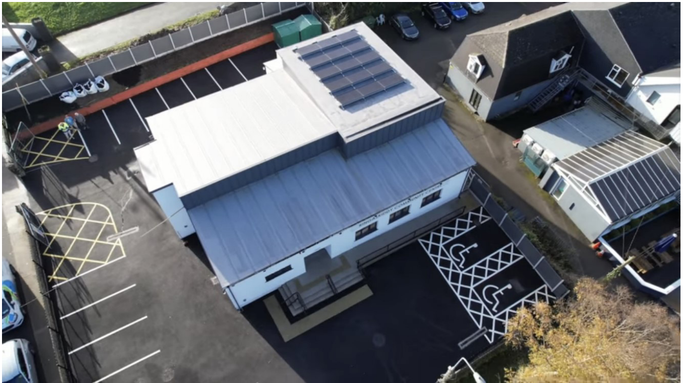
Ringaskiddy Community Hall (New Roof) Town & Village Renewal Scheme
