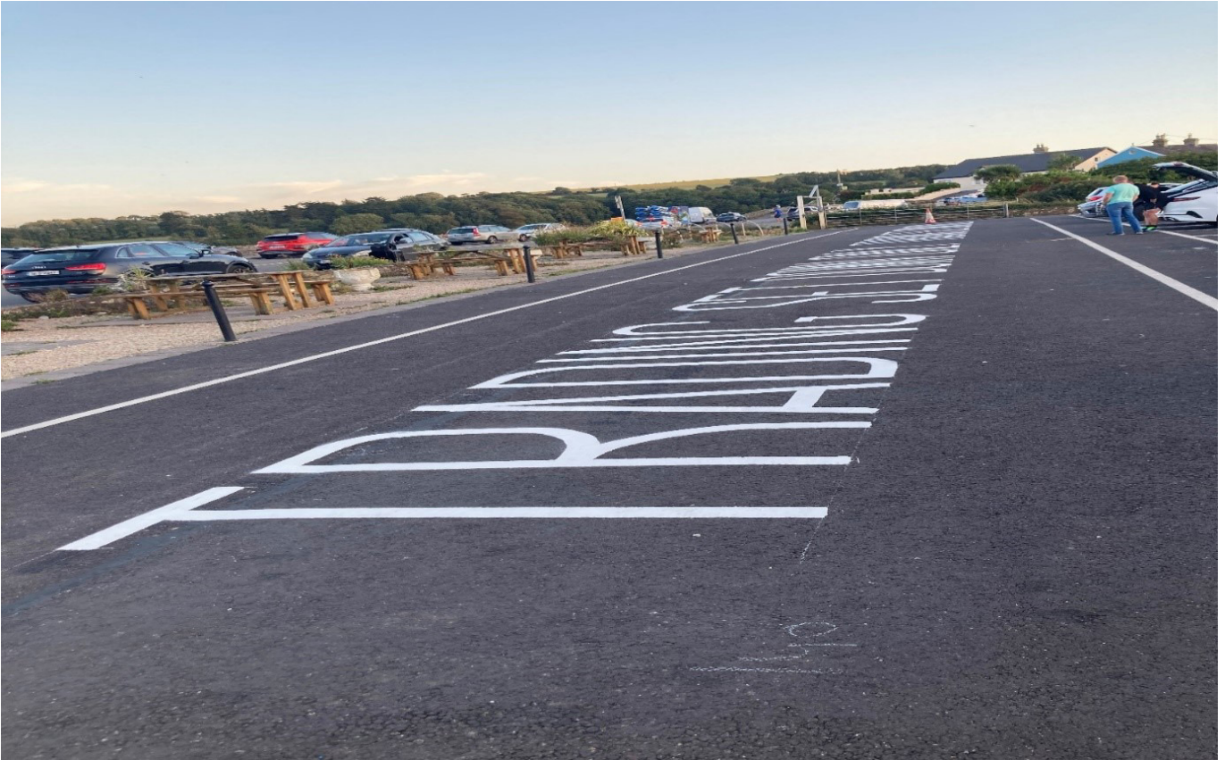
Fountainstown Car Park resurfaced and re-lined, and marked for casual trading
