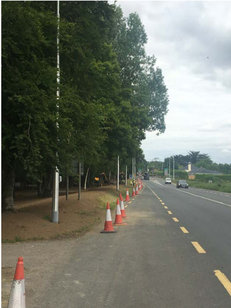
Passive columns erected on the N72 Mallow-Killarney Road
