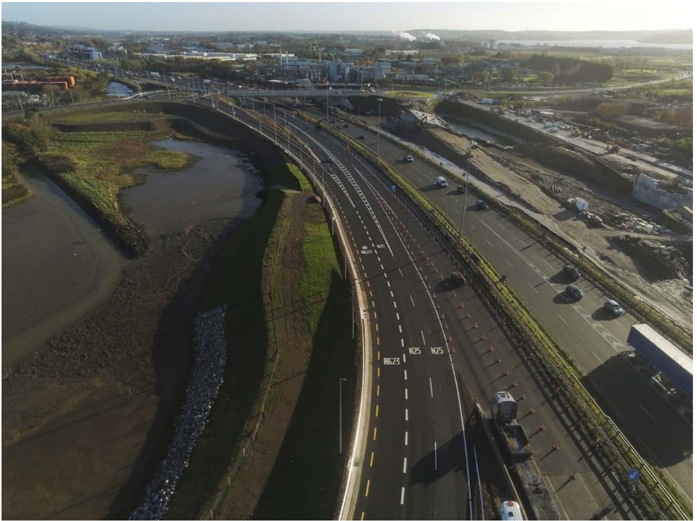
Photo Showing the free flow merge access to the N25 Eastbound from the M8 Southbound, and the free flow access to Little Island via the newly constructed grade separated junction over the N25.
