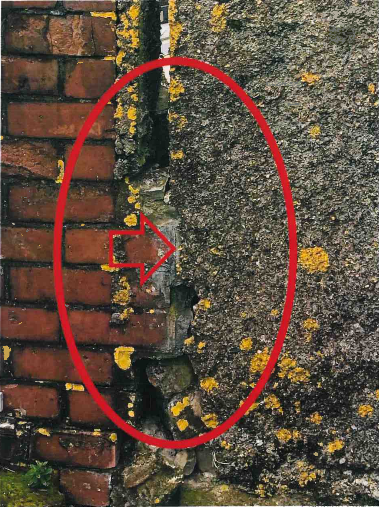
Figure 5 Brick Pier Oct 2023 Detail
