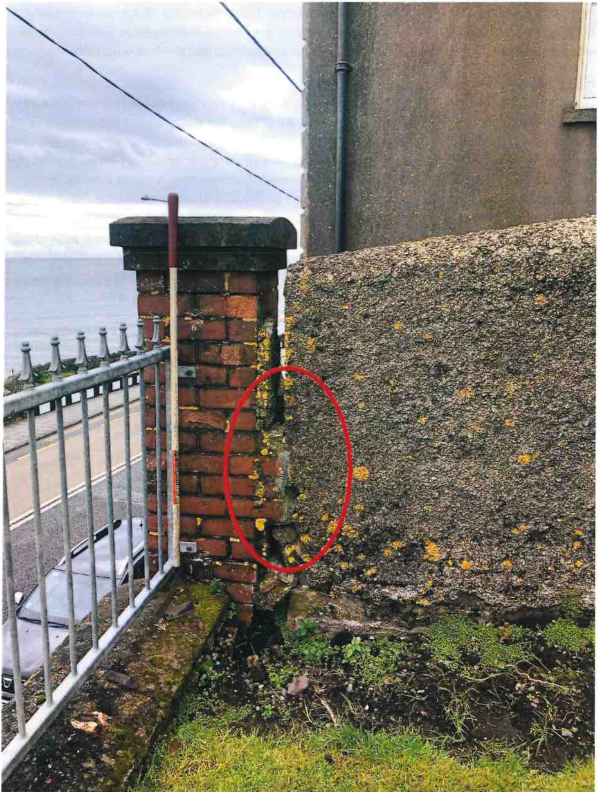
Figure 4 Brick Pier 14th Oct 2022
