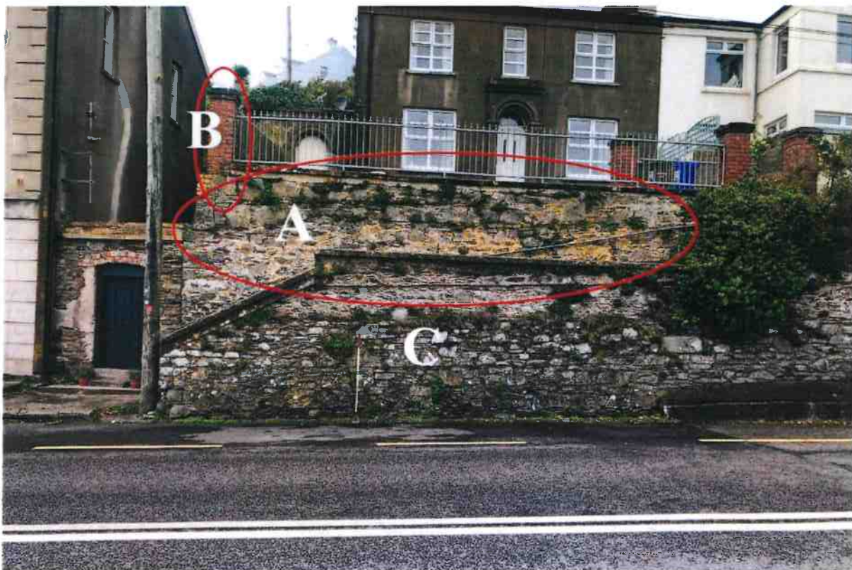
Figure 1 Retaining Wall , Harbour View, Youghal
