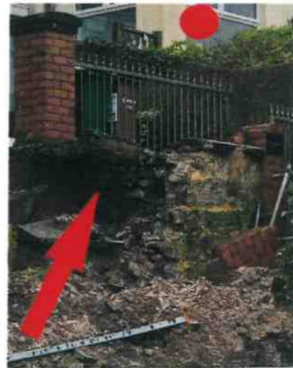
Figure 11 Access Undermined
