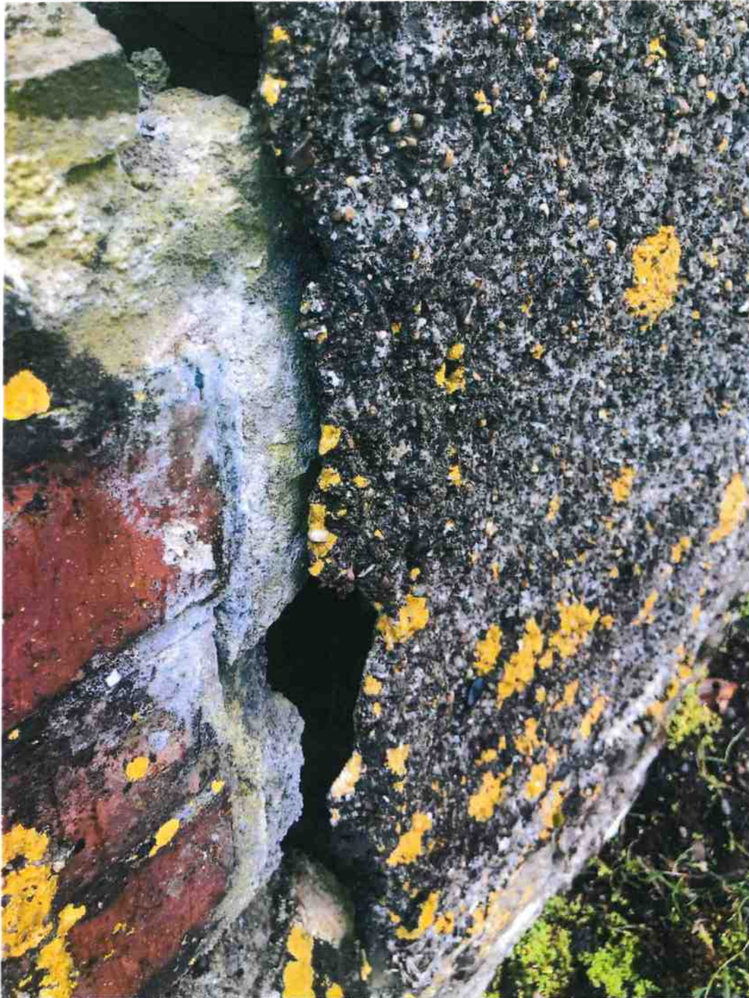
Figure 7 Brick Pier 26 July 2023 Detail: Oblique view
