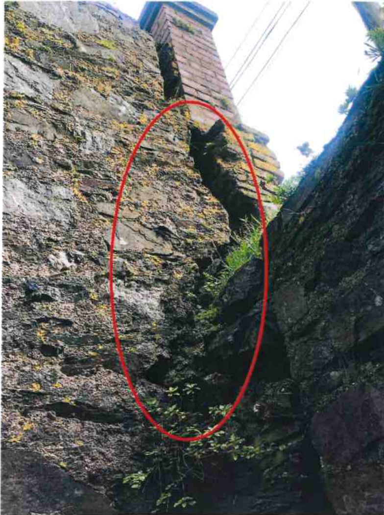
Figure 8 Separation from Return Wall
