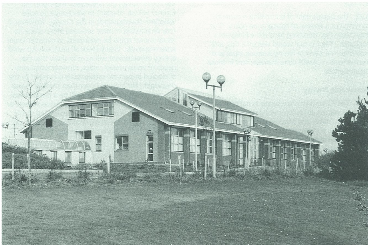
County Council Laboratories, Inniscarra
