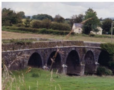
RPS No. 00221 Ballykenly Bridge
