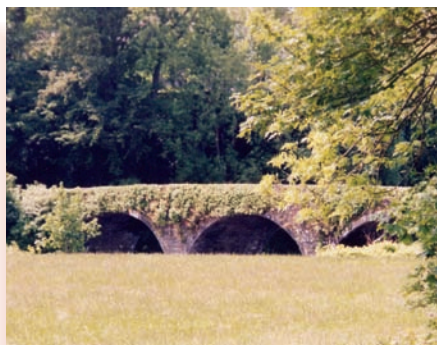
RPS No. 00293 Killavullen Bridge
