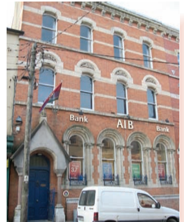
RPS No. 00975 AIB Bank
