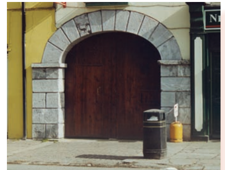
RPS No. 01075 Archway
