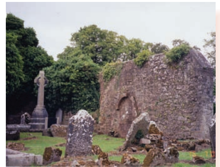
RPS No. 00844 Ballyhay Church (in ruins)
