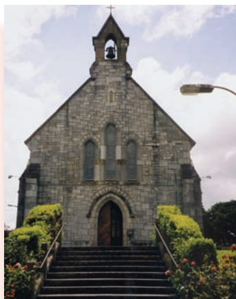
RPS No. 00081 Shanballymore Catholic Church
