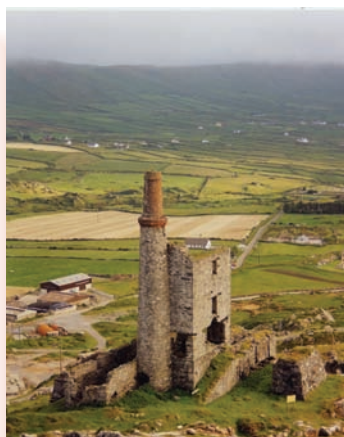
RPS No. 00739 Man-Engine House
