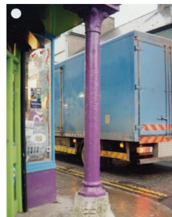
RPS No. 01219 Cast Iron Column outside Duhallow Phone Shop
