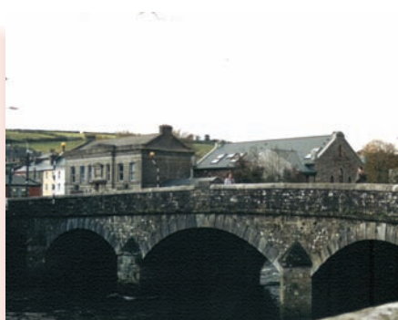
RPS No. 00952 Bandon Bridge
