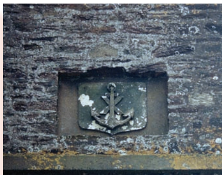
RPS No. 00596 Detail from St. Colman's Church
