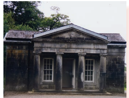
RPS No. 00064 Doneraile Court Country House - Gate Lodge
