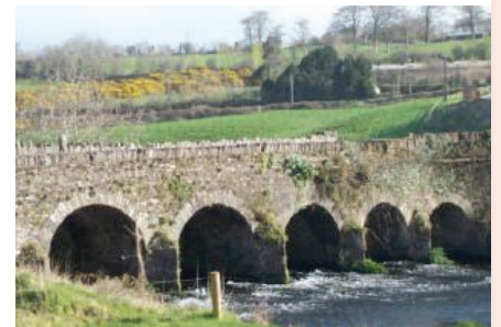
RPS No. 00440 Dripsey Bridge
