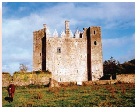
RPS No. 00497 Barryscourt Castle
