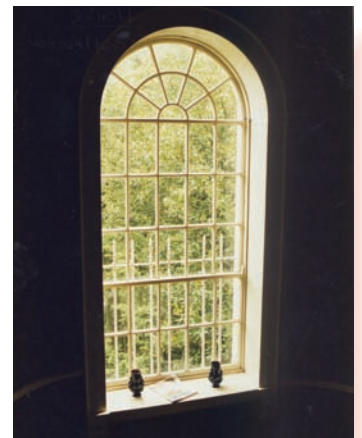
RPS No. 00502 Detail from Ditchley House
