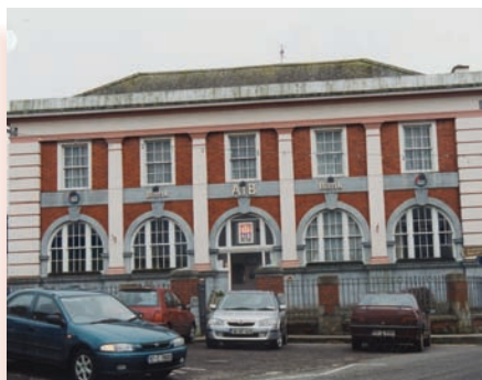
RPS No. 01178 AIB Bank
