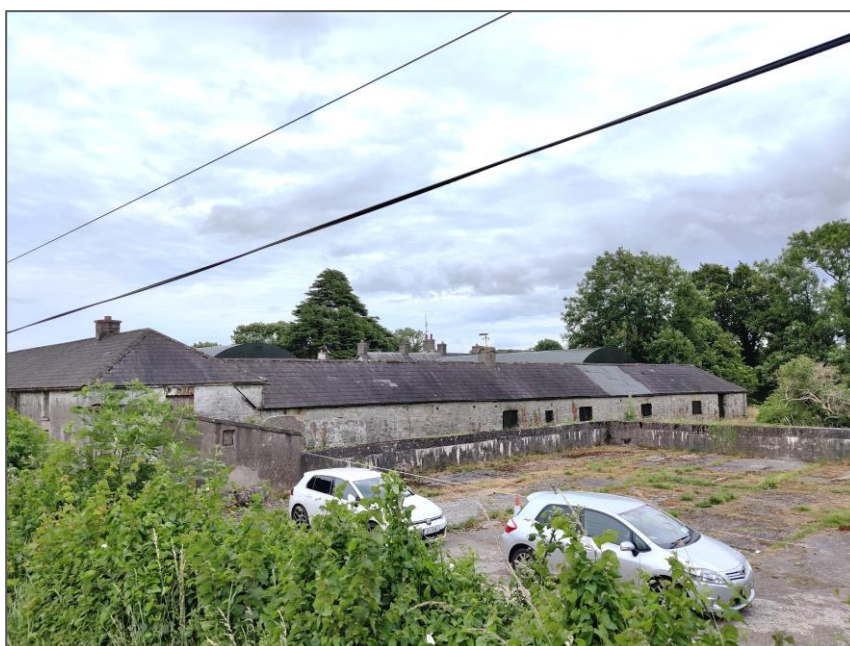
Figure 3-12 - Ballyadam House and outbuildings (03/07/2023).
