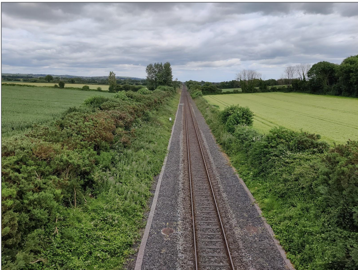
Figure 3-5 - Railway corridor (*RC) viewed from the farm overpass (29/06/2023).
