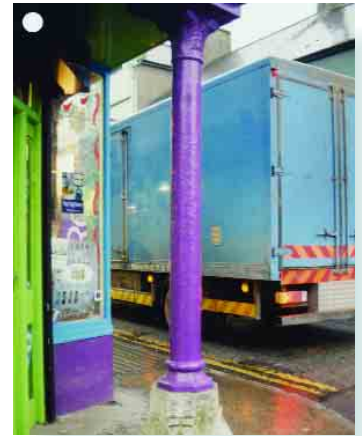
RPS No. 01219 Cast Iron Column outside Duhallow Phone Shop
