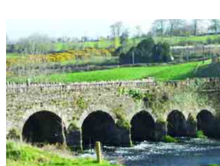
RPS No. 00440 Dripsey Bridge
