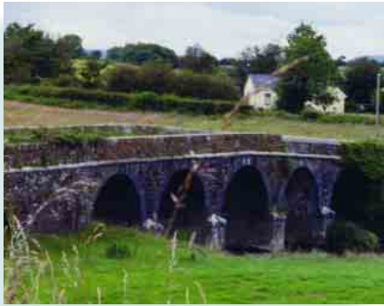
RPS No. 00221 Ballykenly Bridge
