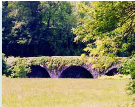
RPS No. 00293 Killavullen Bridge
