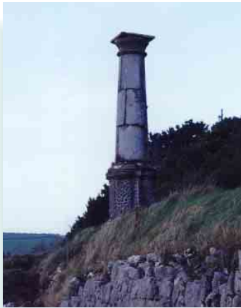
RPS No. 00825 Pedestal
