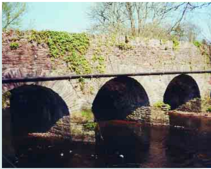
RPS No. 00394 Riverstown Bridge
