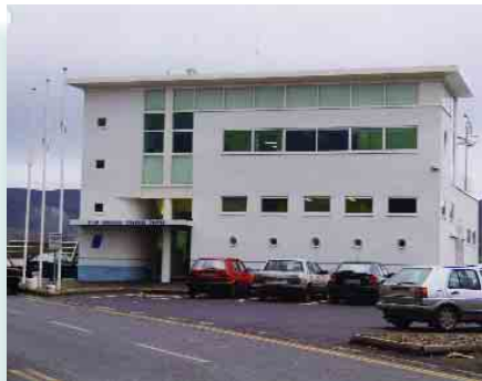
RPS No. 01001 BIM Regional Fisheries Centre
