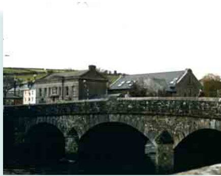
RPS No. 00952 Bandon Bridge
