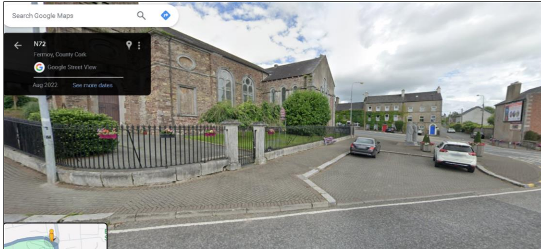
Fig 4 Protected Limestone Kerbing, (Google Maps Streetview)
