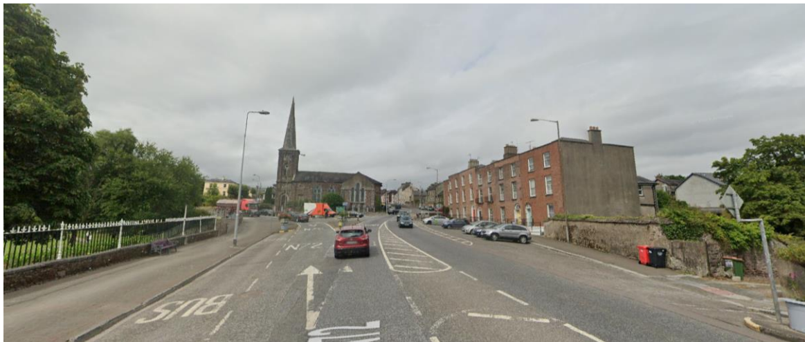
Plate 20— View north towards Christ Church Junction (Google Maps Street View, image date July 2022)
