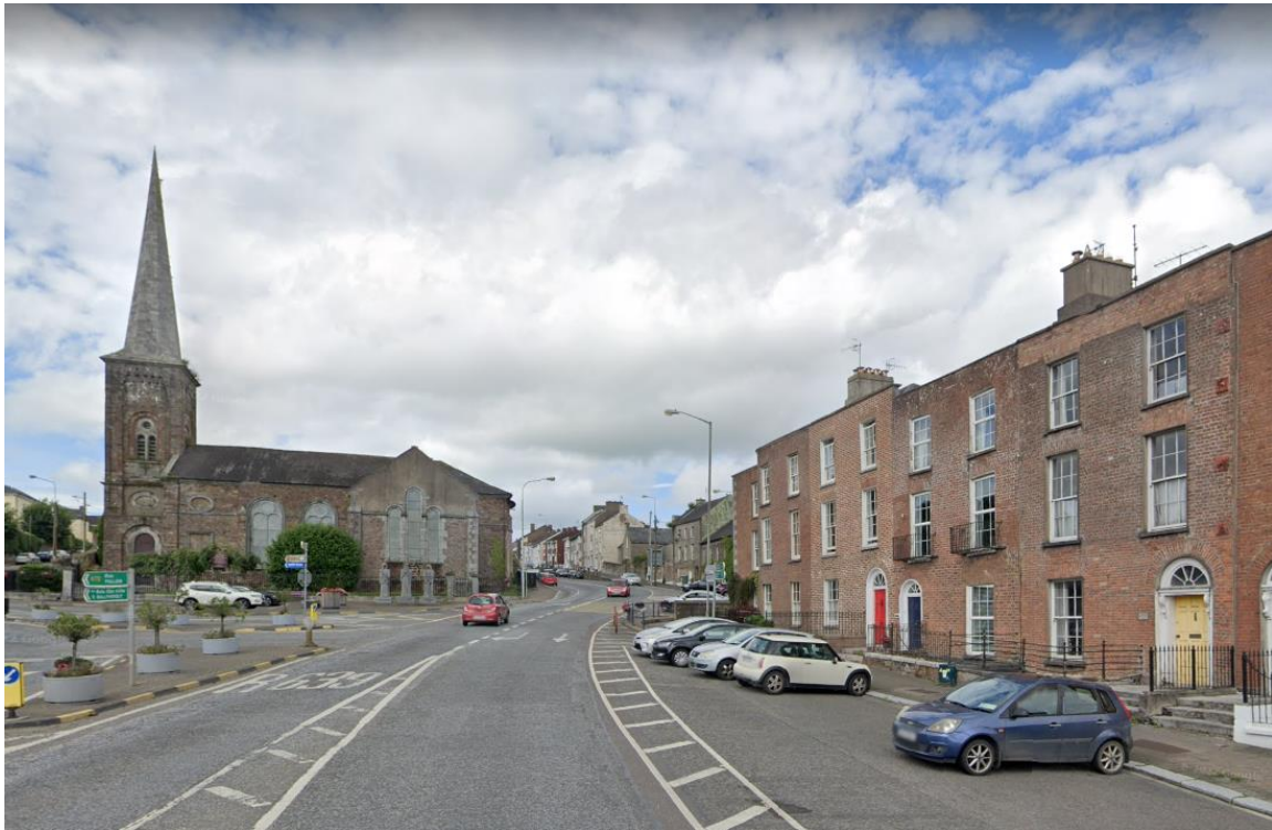
Plate 1— Christ Church (RPS ID: 2,231) on left of image with 1-4 St. James' Place (RPS IDs: 2241-4) on right. (Google Street View, image capture date August 2022)
