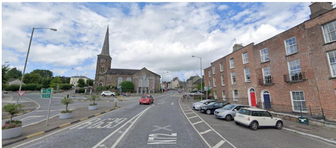
Plate 21— View of N72 Christ Church Junction looking north (Google Maps Street View, image date August 2022)
