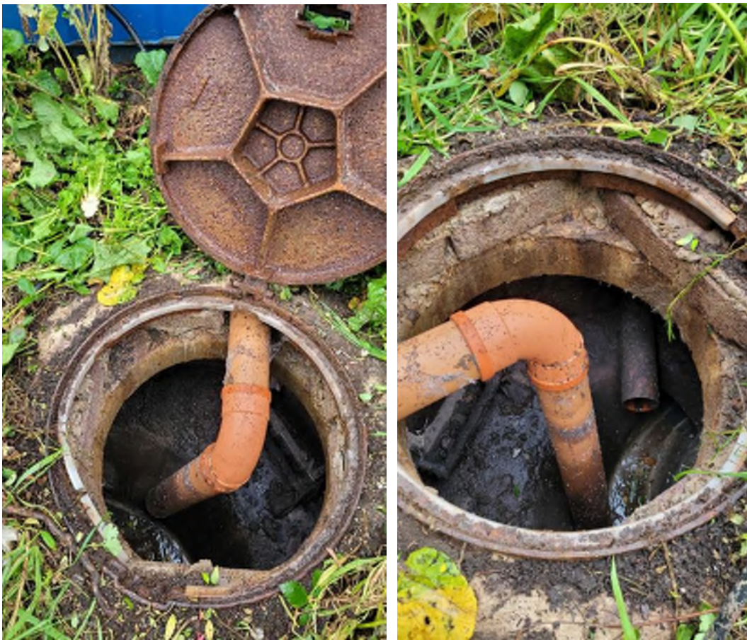
Previously covered foul manhole north of no. 19
