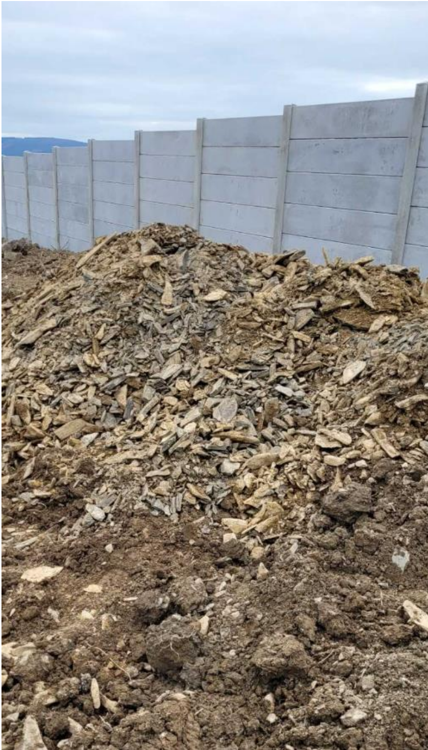
Material excavated from trial hole to rear of site of no. 19
