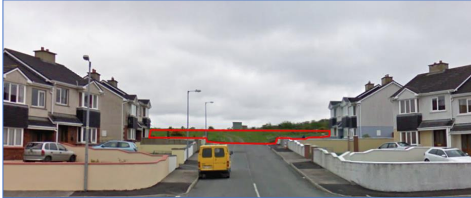
Figure 2: View of the site from the existing access road.
