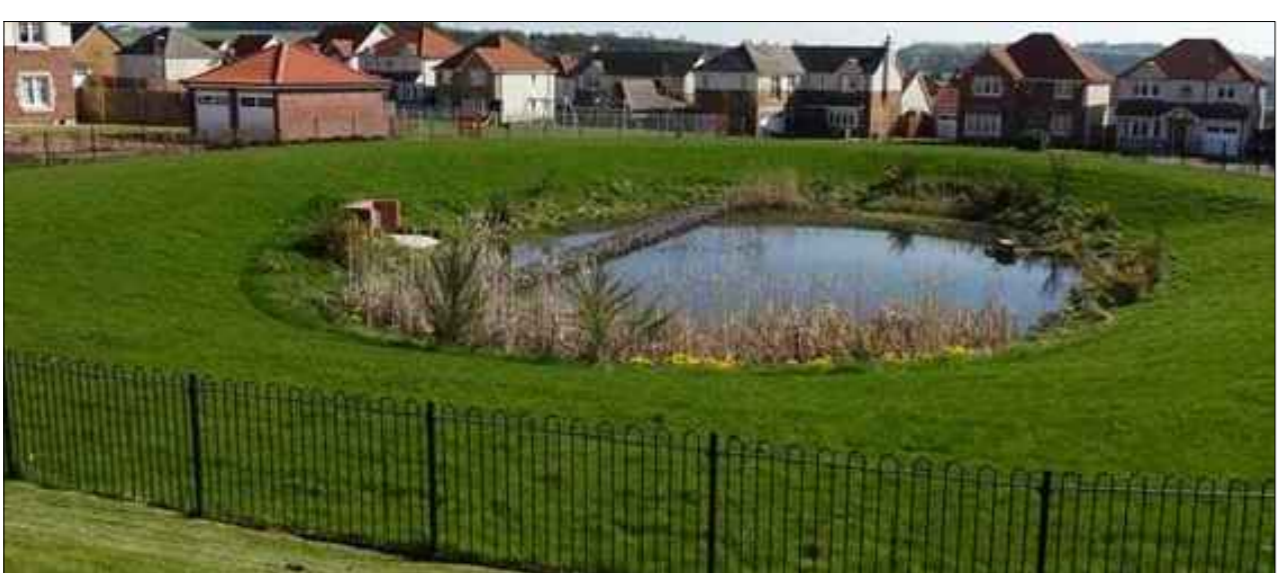
1. Example of Water Retention Pond, to be graded and naturally planted on banks.
