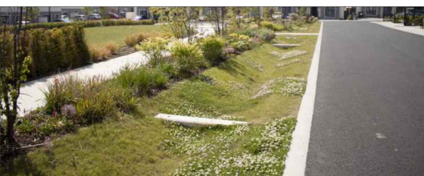
2. Example of Grass Swale, with proposed grading from road into proposed filter drain.
