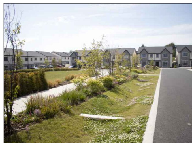
3. Example of Grass Swale along Roadside.
