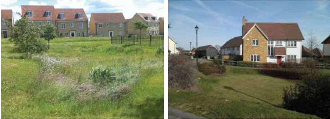
Figure 7: Examples of detention basins by Peterborough City Council in the UK (CIRIA SuDS Manual C753)
