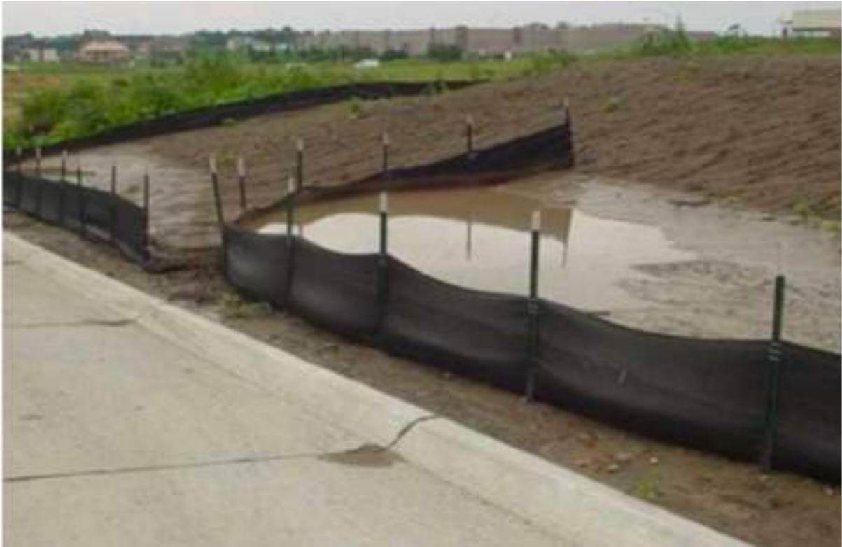
Figure 11. Typical silt fence arraignment.
