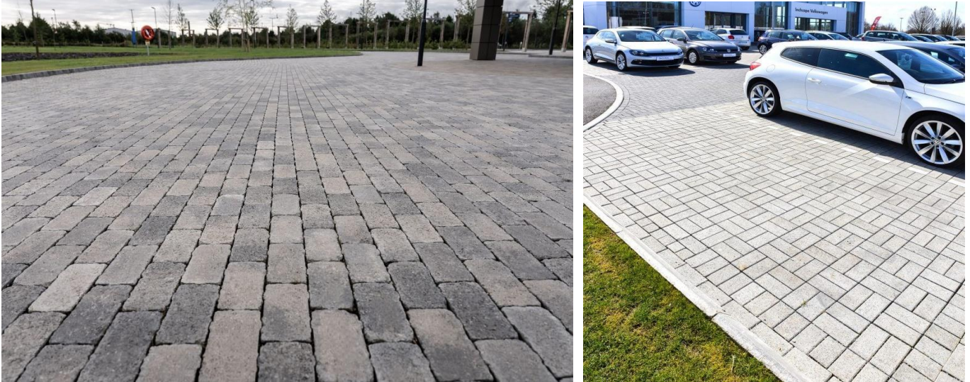
Figure 17 Example of permeable block paving system
