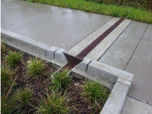
Figure 19 Example of drainage within concrete footpath
