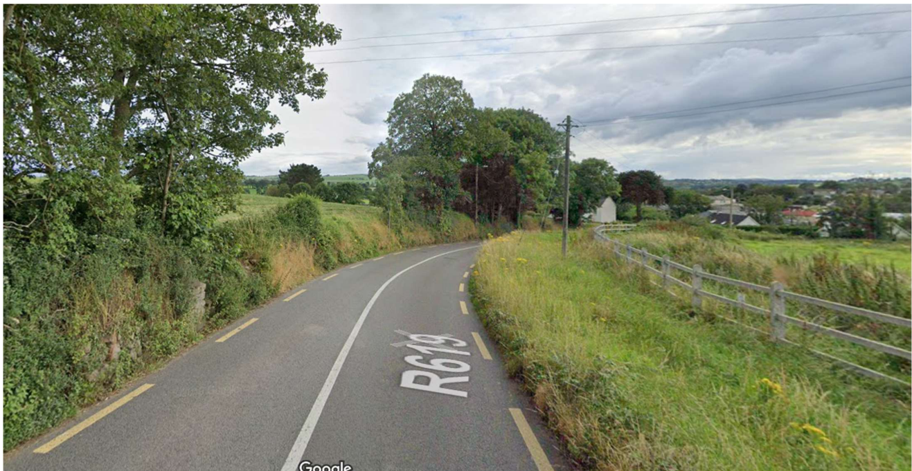
Figure 4 - Construction Site Access
