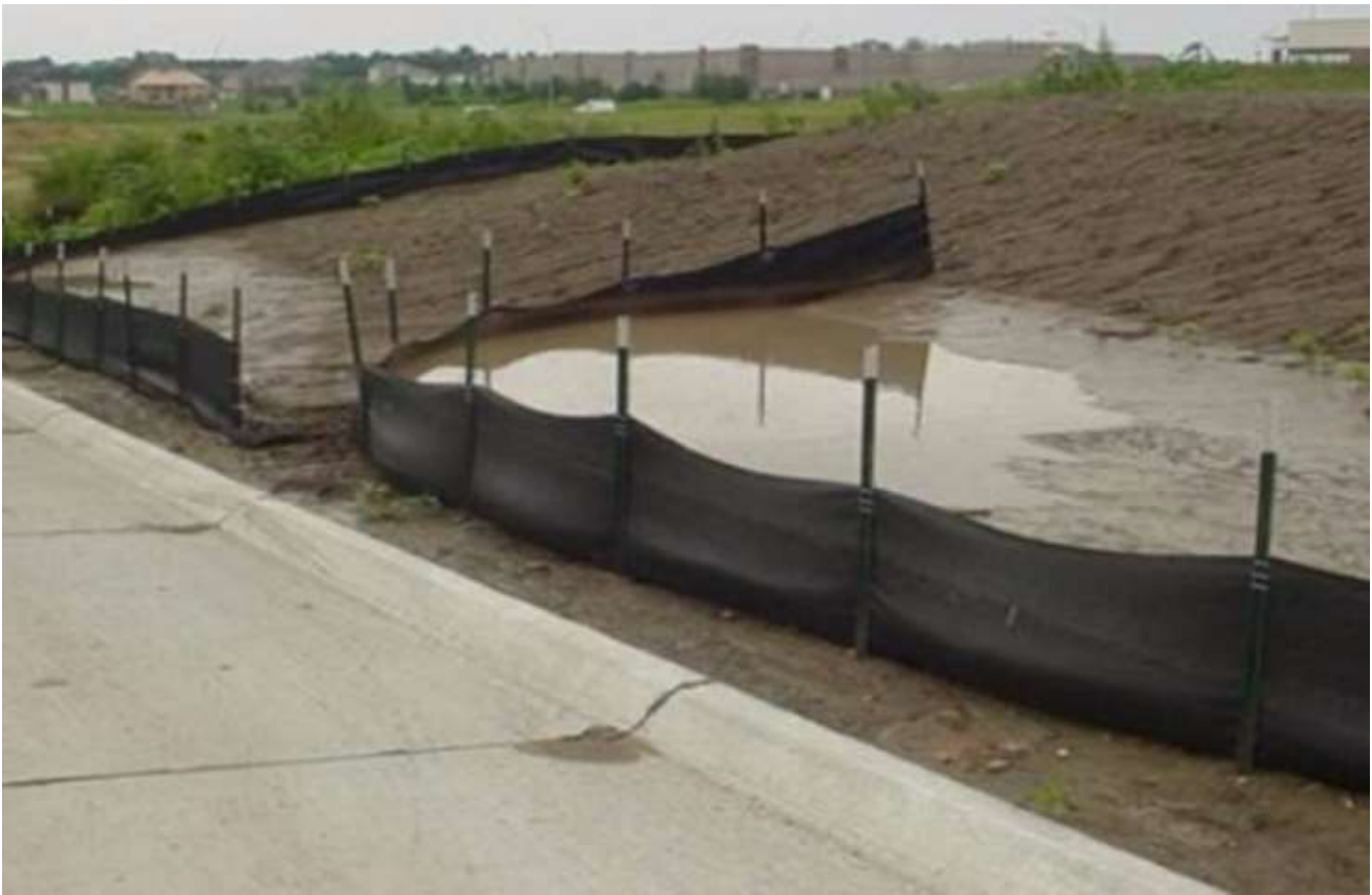
Figure 5 - Typical Silt Fencing Arrangement
