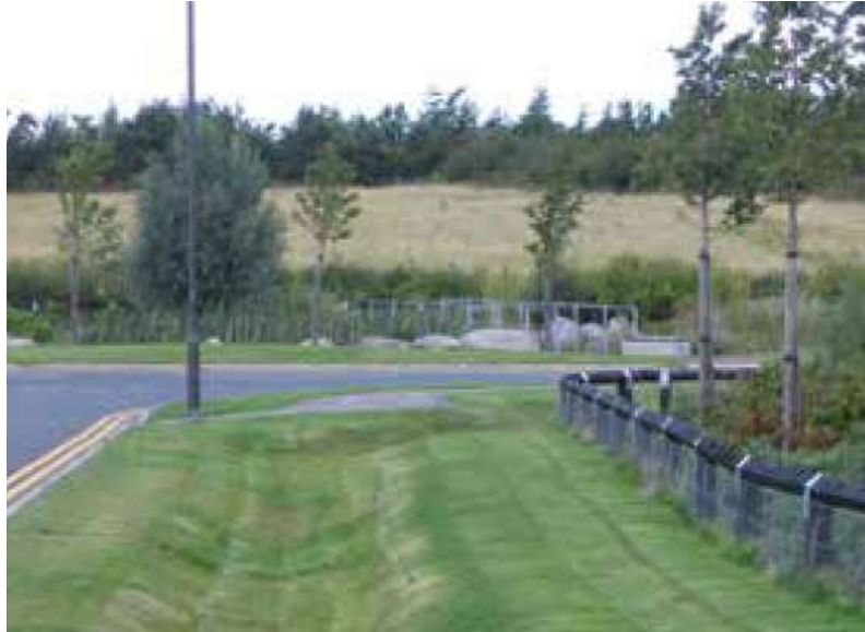
Figure 8: Example of roadside swale from the CIRIA SuDS Manual (C753)
