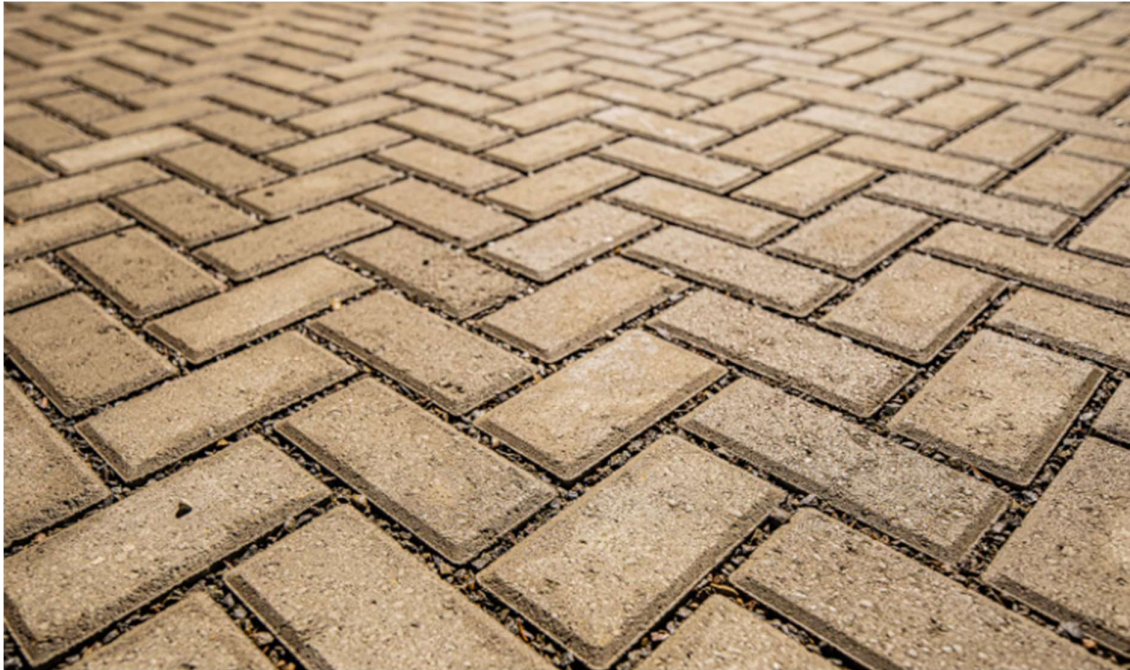
Figure 9: Example of permeable paving.
