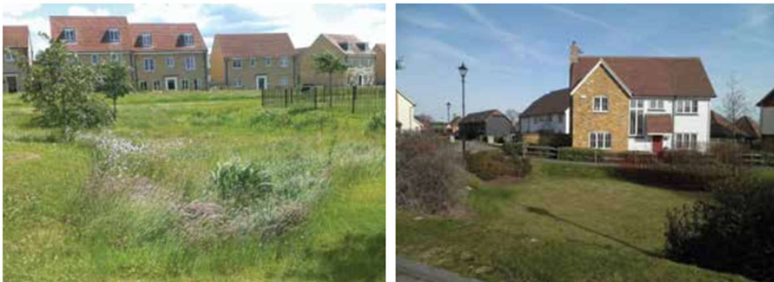
Figure 6: Examples of detention basins by Peterborough City Council in the UK (CIRIA SuDS Manual C753)
