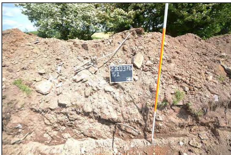
Photograph 6: The modern building debris mixed with the topsoil in the middle to south of Test Trench 1.
