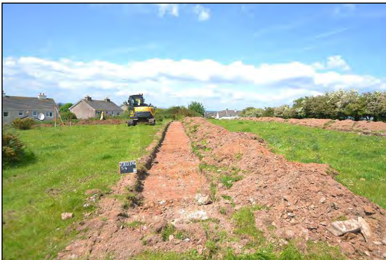
Photograph 15: Test Trench 4 From the south.
