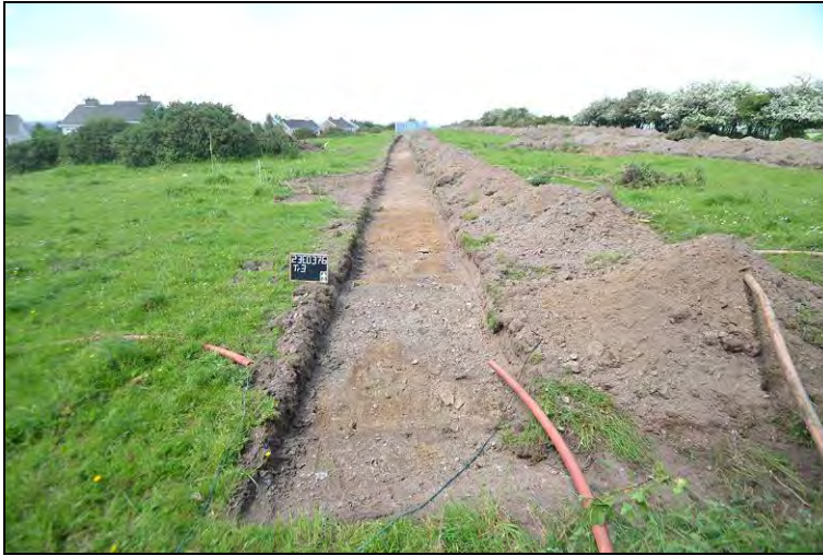
Photograph 14: Test Trench 3 From the south.
