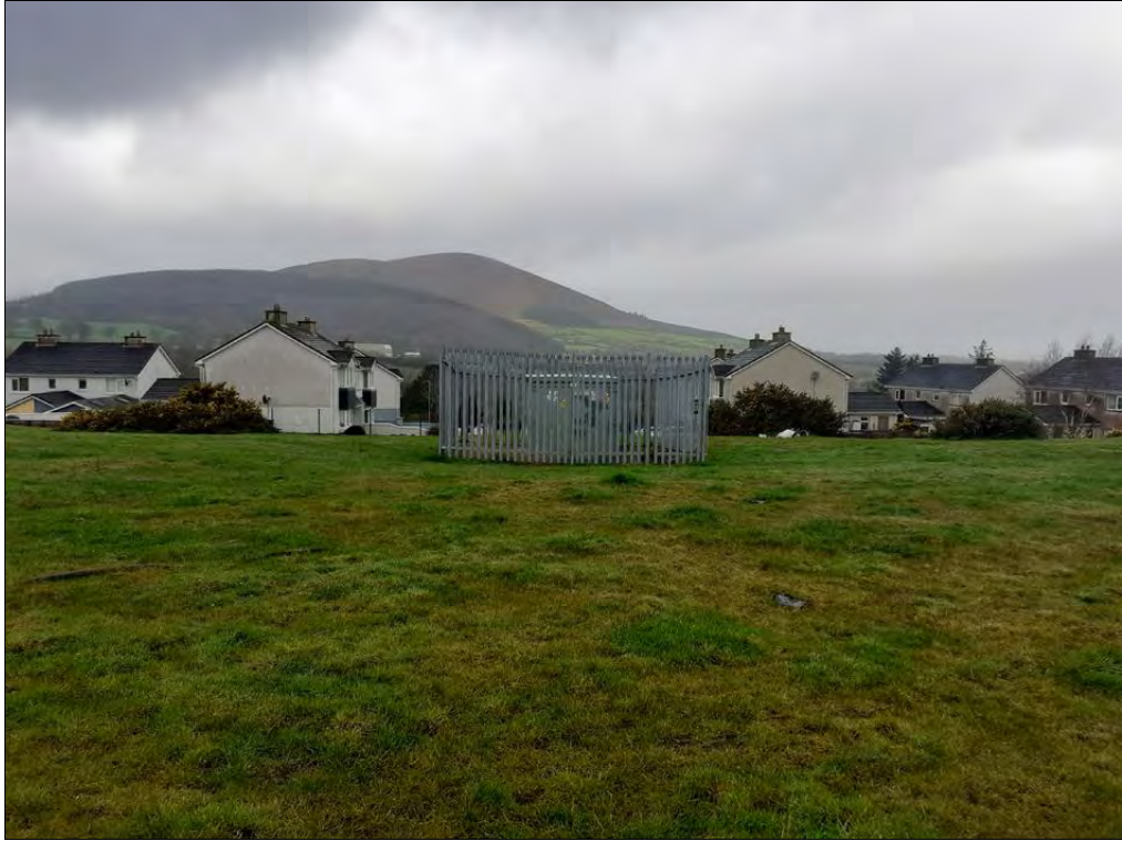
Plate 3. Transformer box and surrounding steel palisade fence, looking west.
