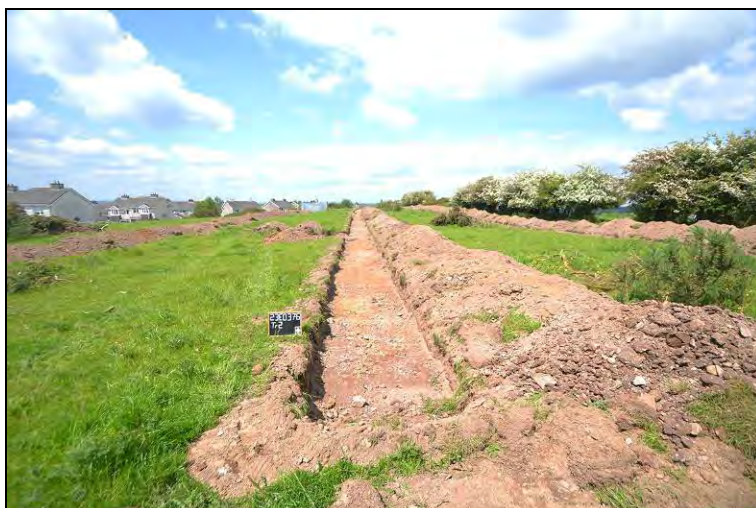
Photograph 7: The southern extent of Test Trench 2.
