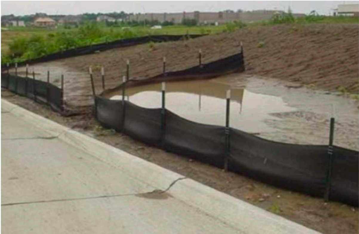
Figure 7. Typical silt fence arraignment.
