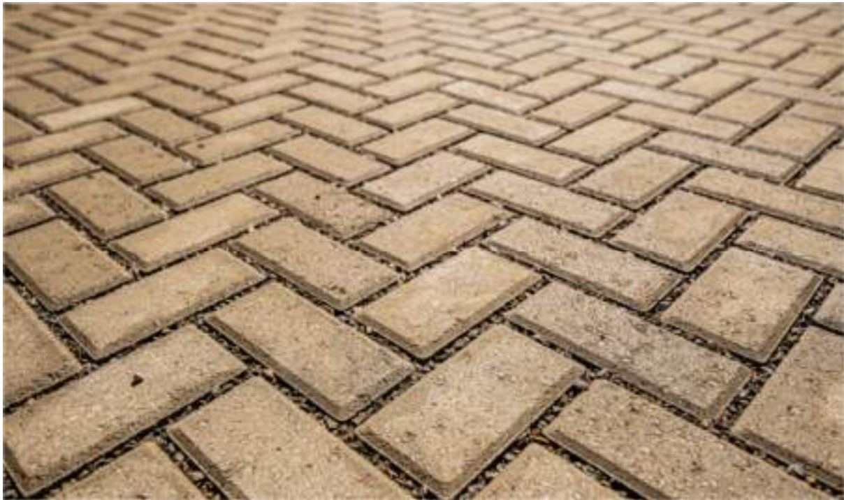
Figure 9: Example of permeable paving
