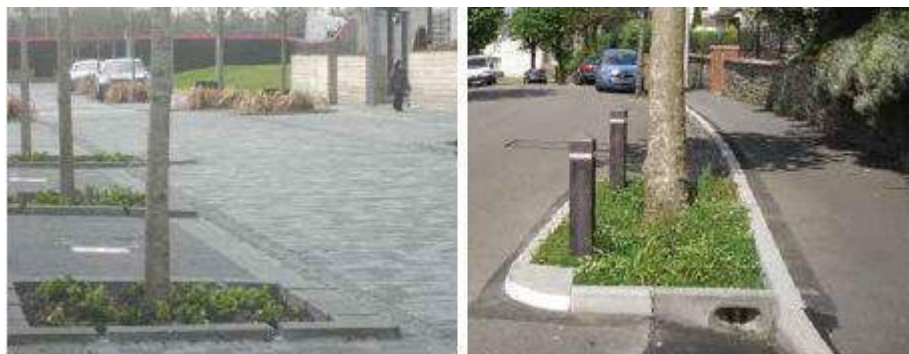
Figure 10: Examples of tree pits in isolated green planters from the CIRIA SuDS Manual
