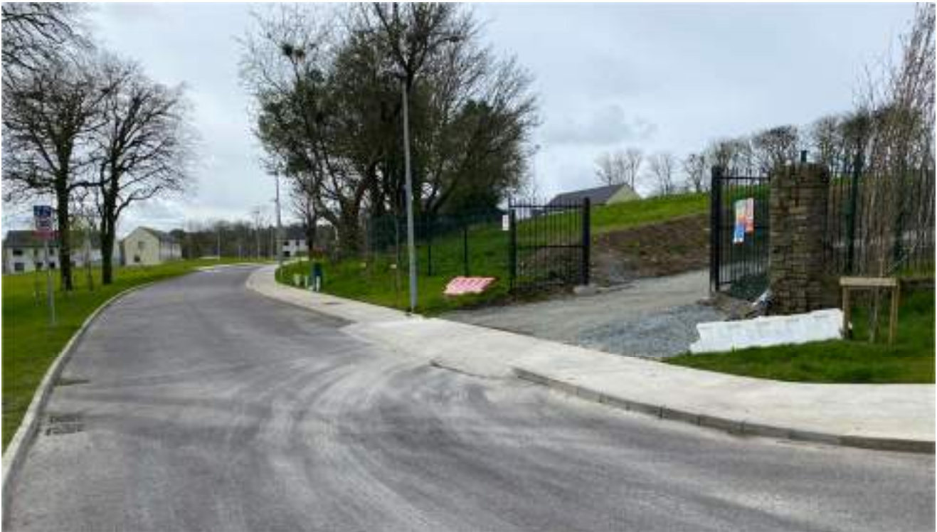
Figure 4 - Construction Site Access
