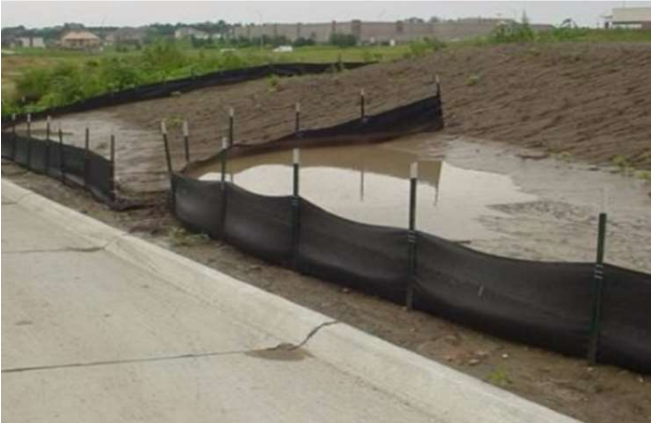
Figure 5 - Typical Silt Fencing Arrangement
