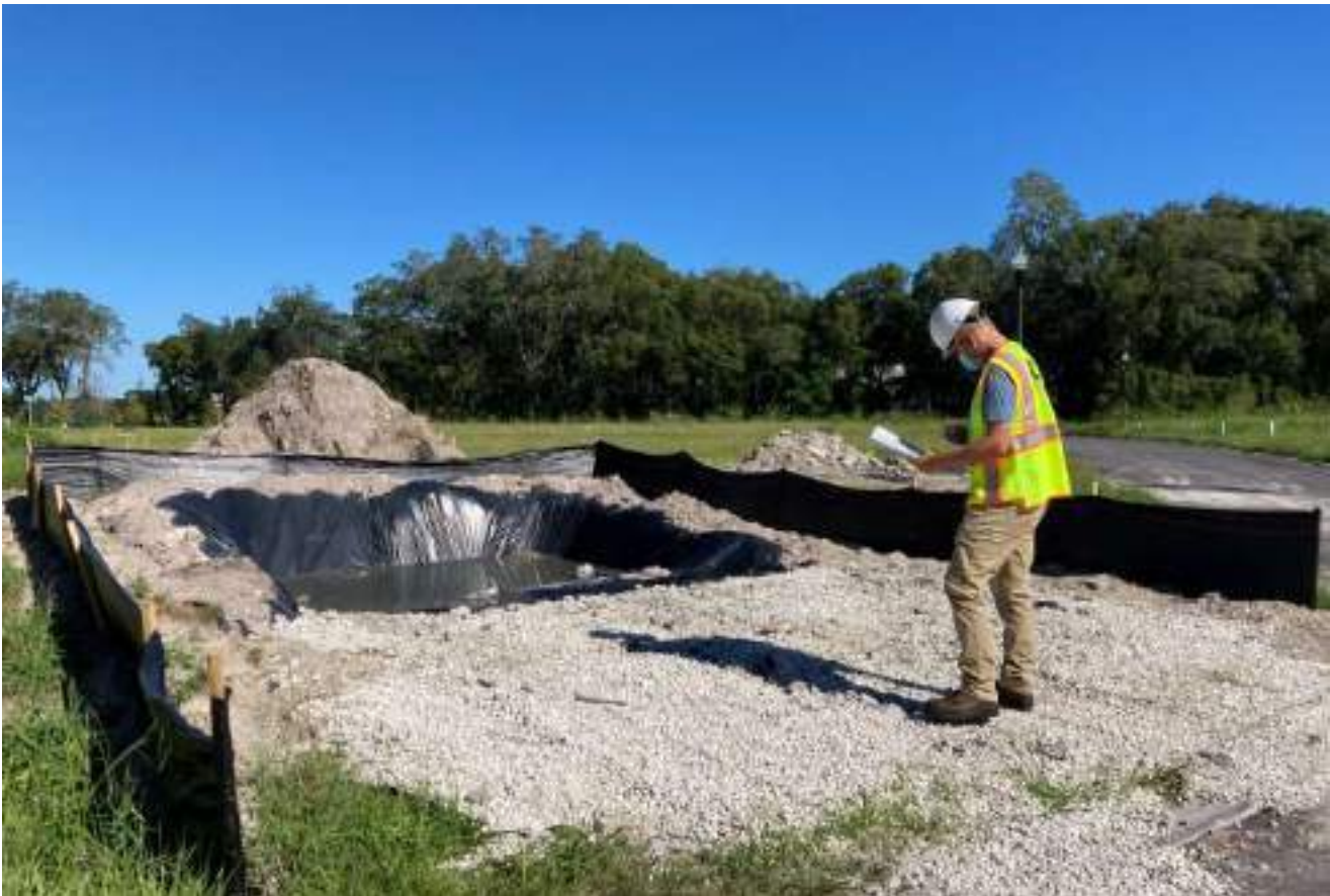
Figure 7 - Concrete Truck Washout Area with Impermeable Liner
