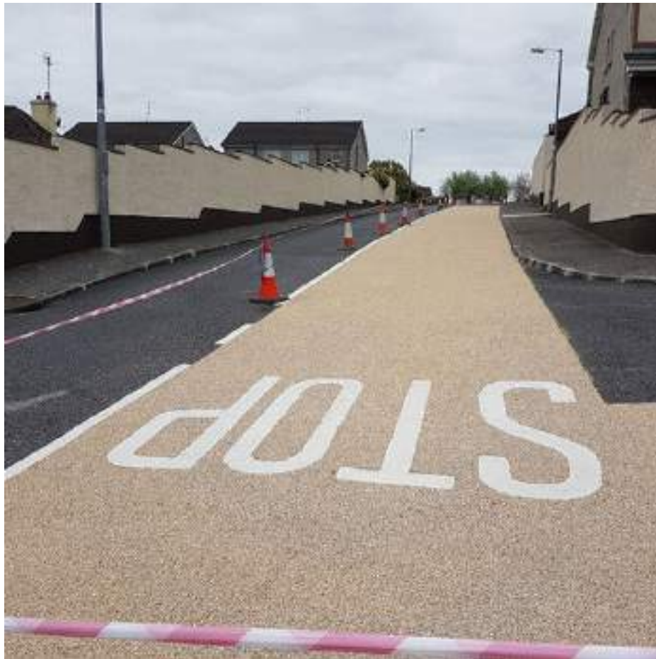
Figure 7: High friction/Anti-skid surfacing on a steeply sloped road approaching a junction.
