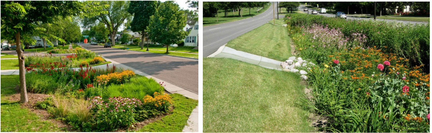
Figure 7 Example of two Rain Garden Bio Swales
