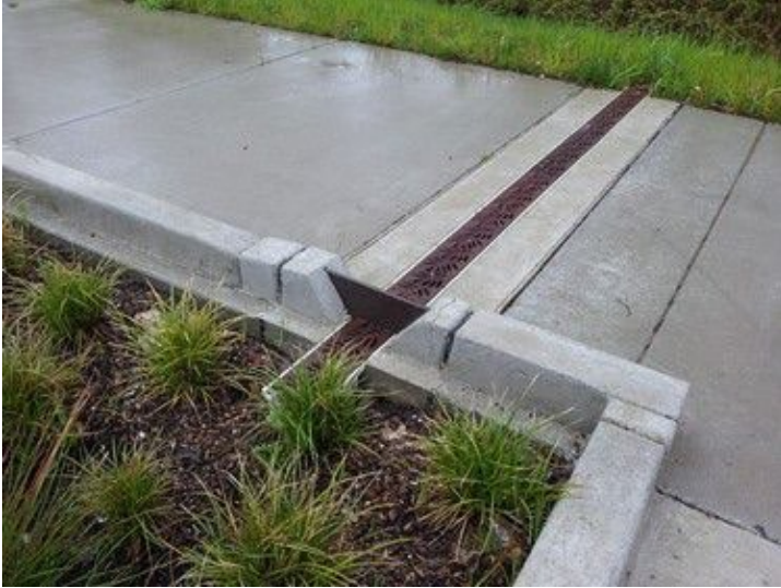
Figure 23 Example of drainage within concrete footpath
