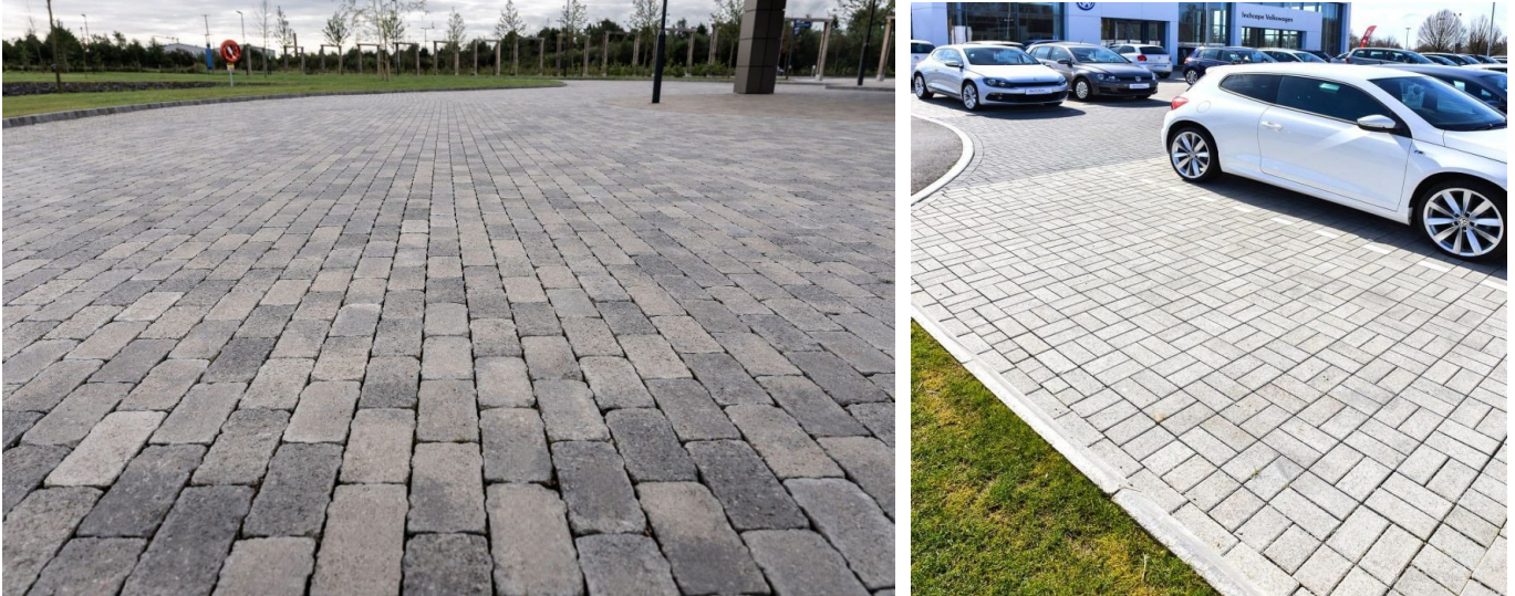
Figure 21 Example of permeable block paving system
