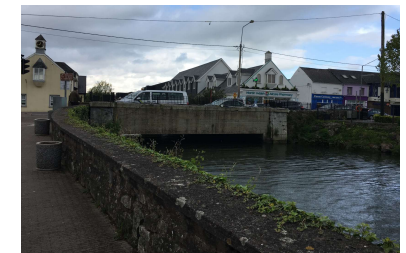
Cork Road bridge
