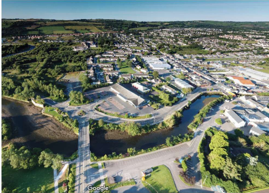
Aerial view of the site
