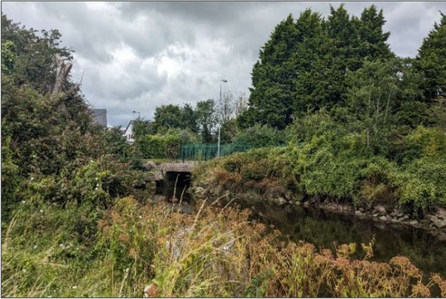
Plate 4.11 View of the northern bank of the Owenboy within the red line boundary of the proposed project. (Bridge to tidal back channel in the centre middle ground).
