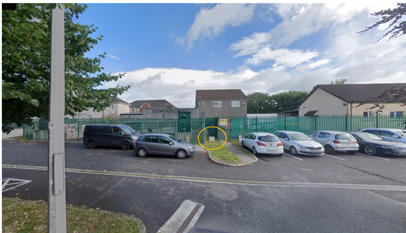
Figure 2-3 - Potentially Undergrounded ESB Cable
