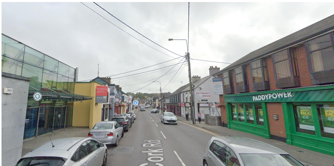
Figure 2-2 - Main Street Electricity Pole
