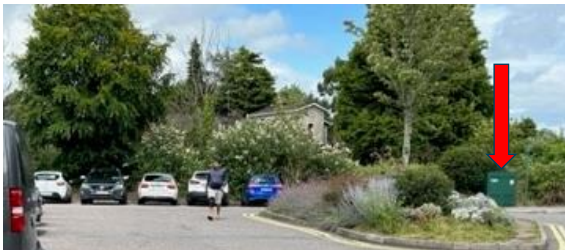
Figure 2-6 - Existing ESB Cabinet in Line of Proposed Parking
