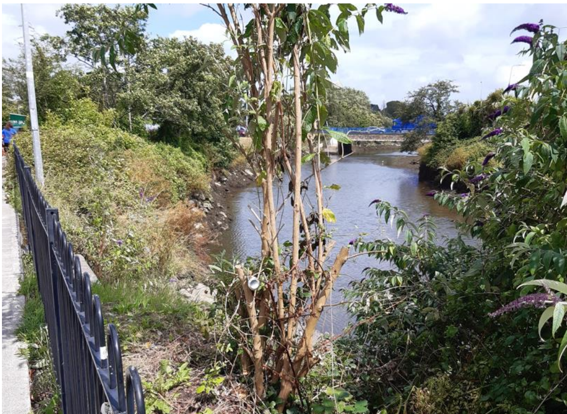
Figure 2-5 - Existing Railing and River Embankment
