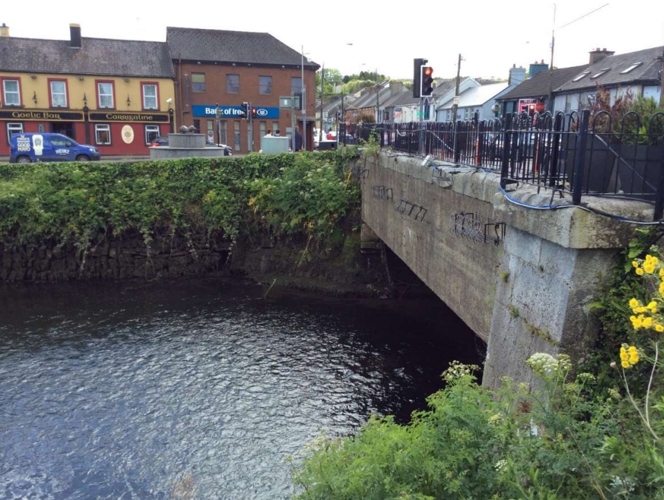
Plate 6: Road bridge over River Owenabue at western site boundary, looking S.
