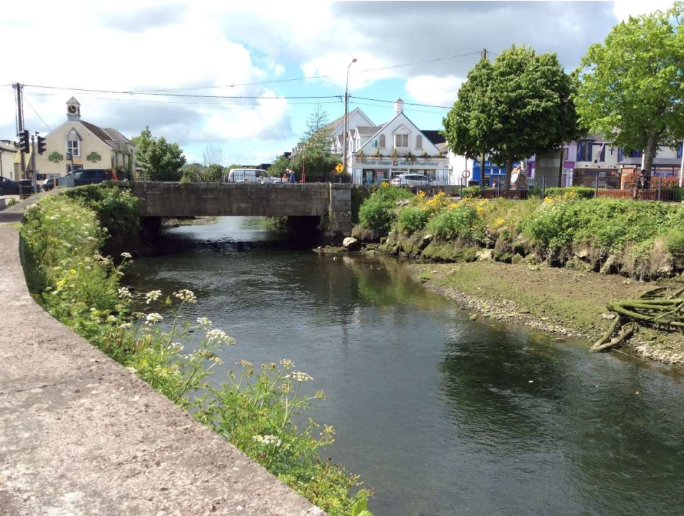
Plate 7: Owenabue River from south bank, looking W.
