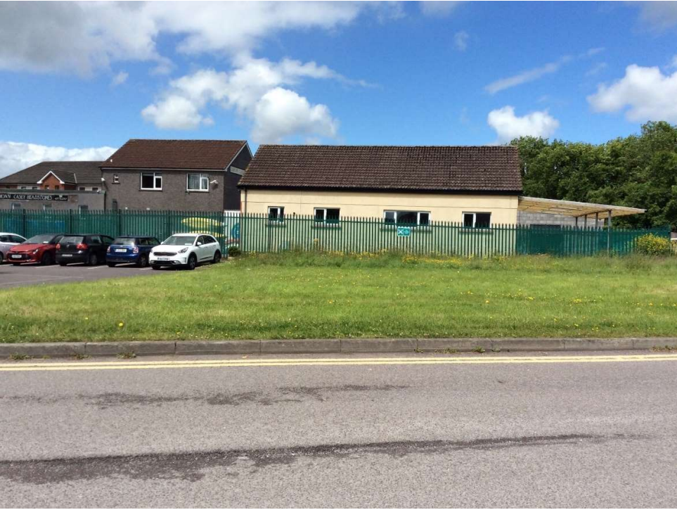
Plate 3: Landscaped green area at NE side of Proposed Development site, looking N.
