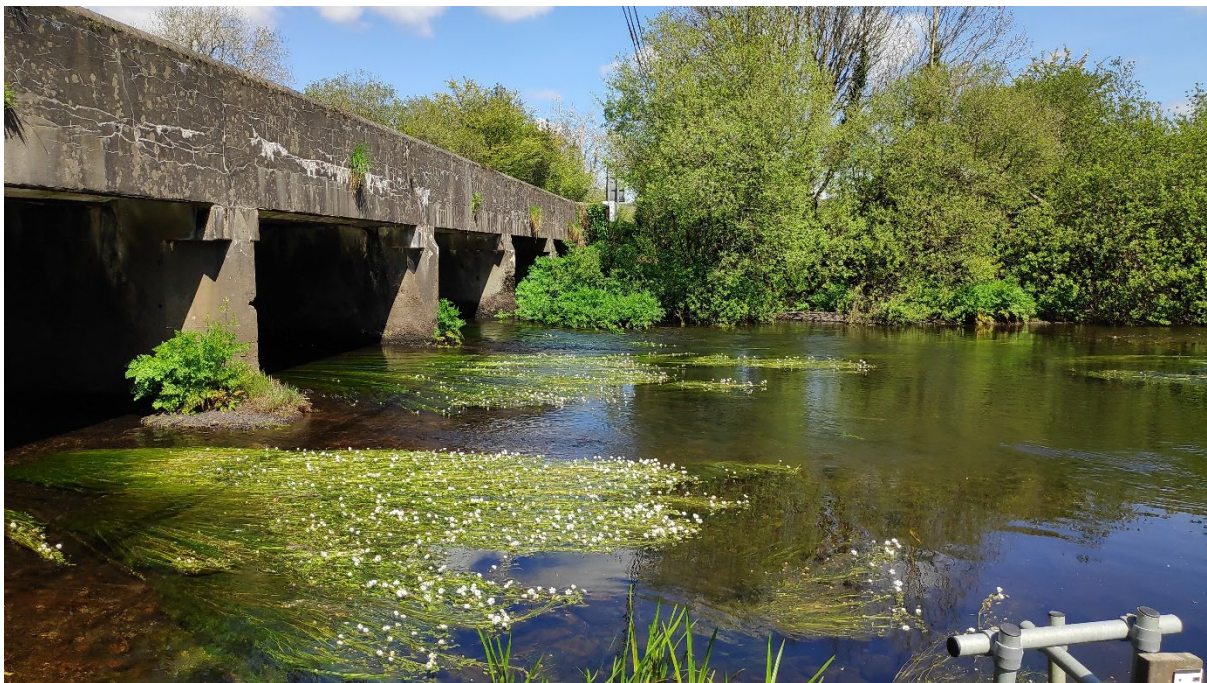
Plate 3.2 Section D immediately downstream of Ardcahan Bridge
