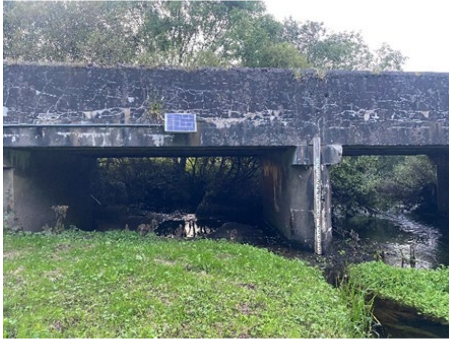
Plate 2-3: View of westernmost arch from downstream location
