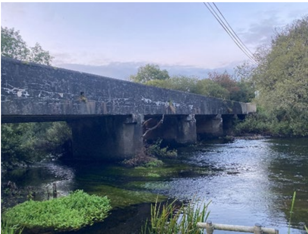
Plate 2-2: View of easternmost arches from downstream location
