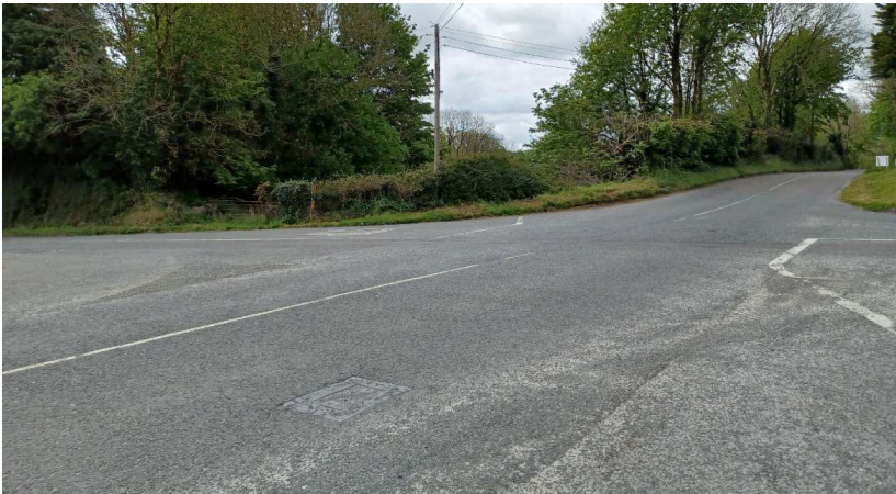
Figure 3 View from North West Looking North East
