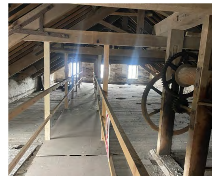
Interior of Steam Mill
