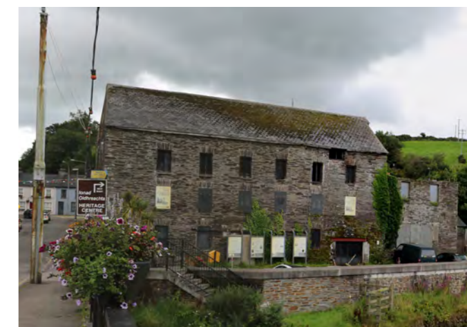
North Elevation of Steam Mill
