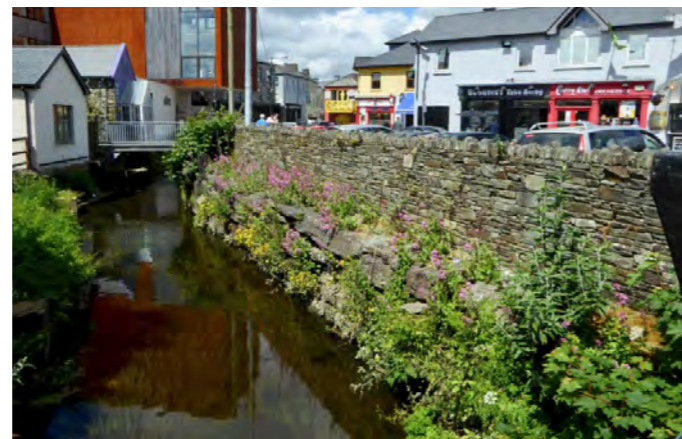
Caol Stream before flood defence works
