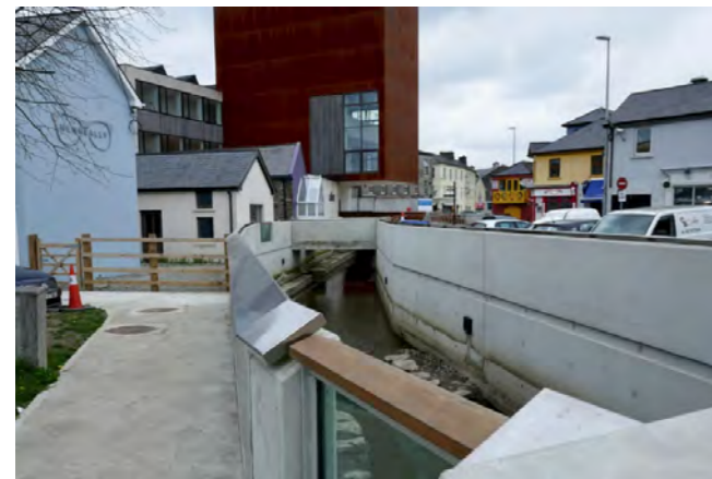
Caol Stream after flood defence works
