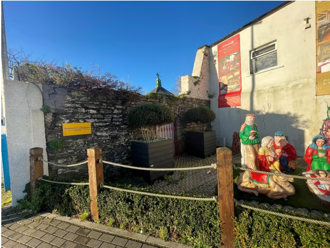
Photograph No. 5 – Southwestern return wall
