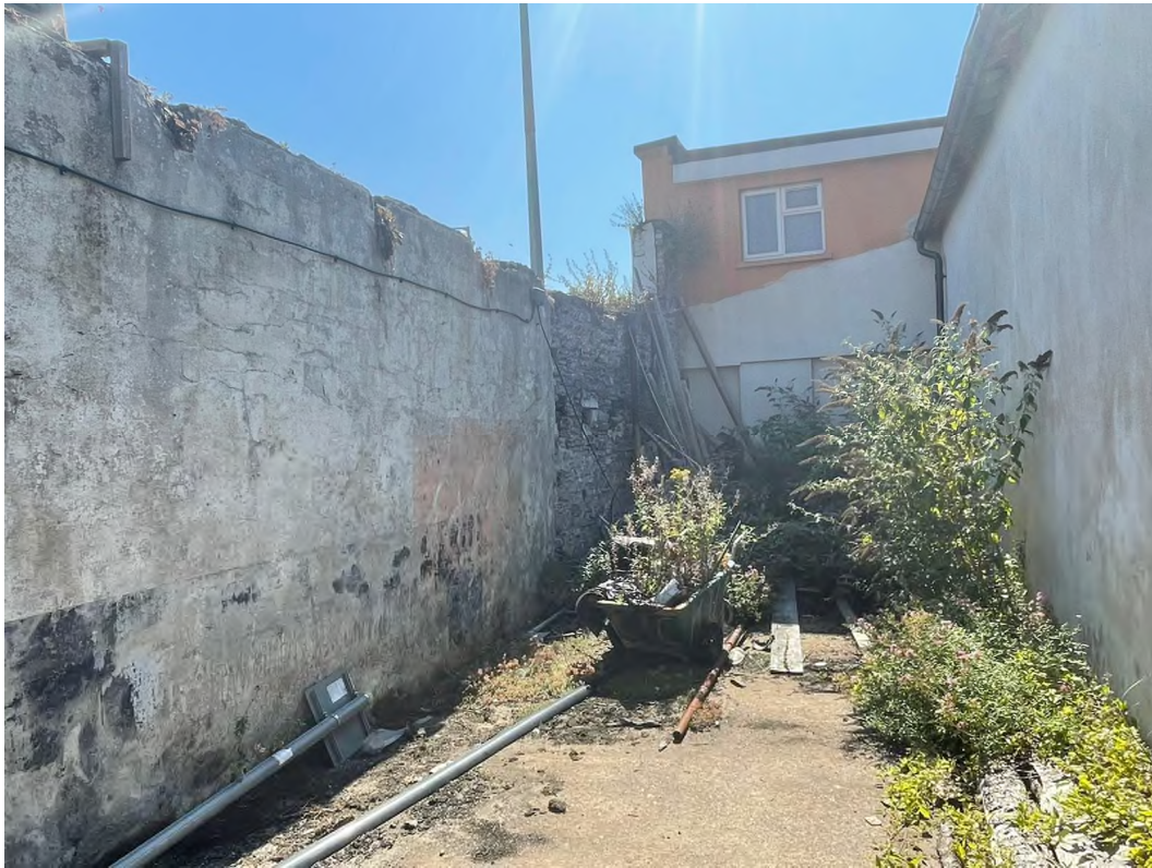
Photograph No. 1 – Internal Face of Wall
