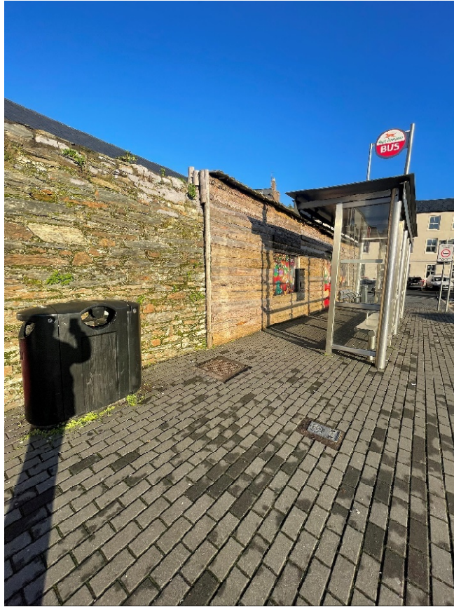
Photograph No. 3 – Long Quay End of Wall
