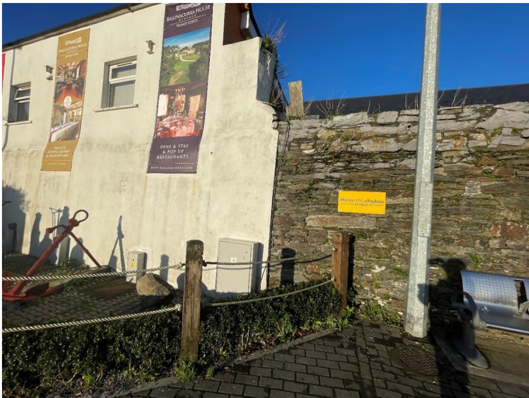
Photograph No. 2 – Short Quay End of Wall
