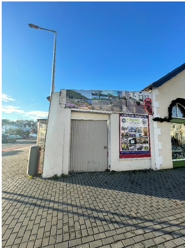
Photograph No. 4 – View from Long Quay
