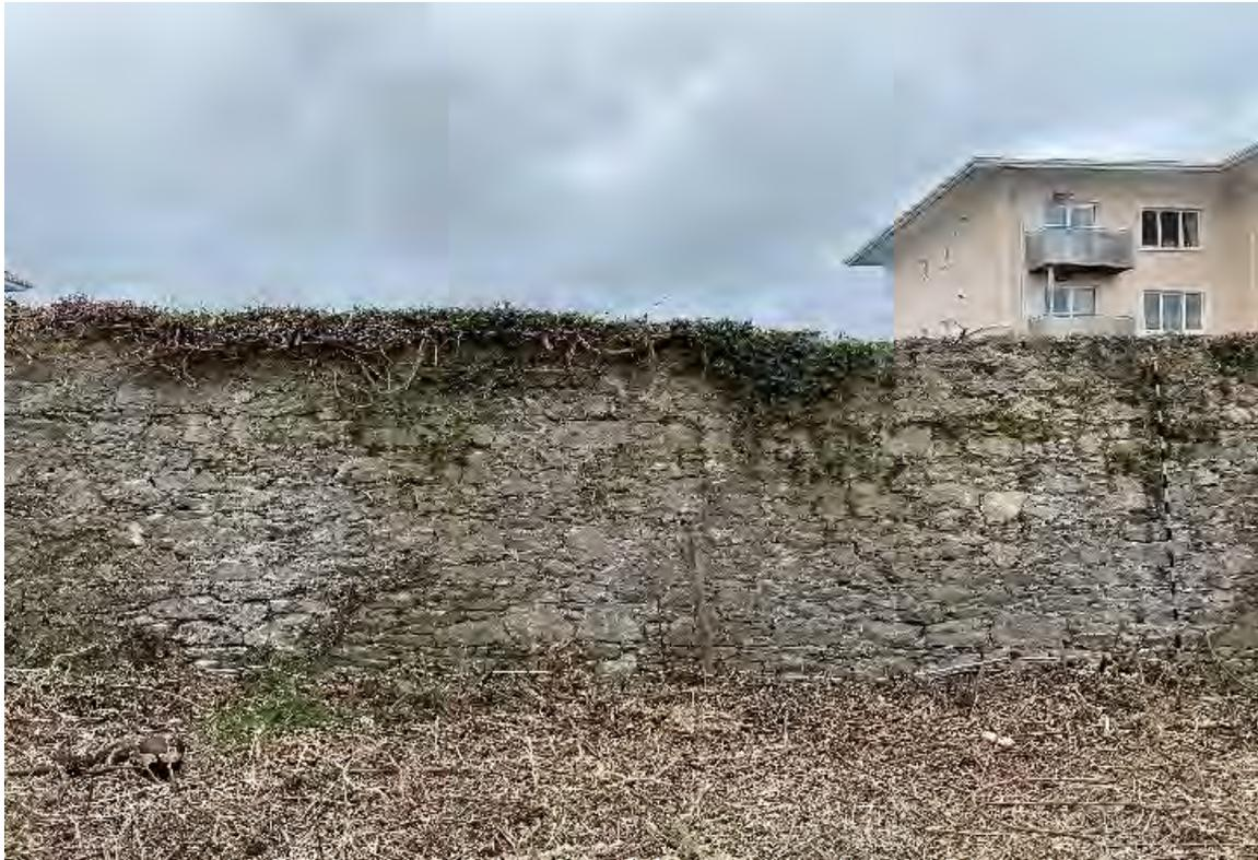
*Figure 17. Sample image of wall showing Central section of north wall. Generally good condition with areas of repointing in lime mortar required as well as ivy treatment and subsequent domed lime mortar capping.*
