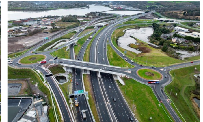
Dunkettle Interchange – Looking West
