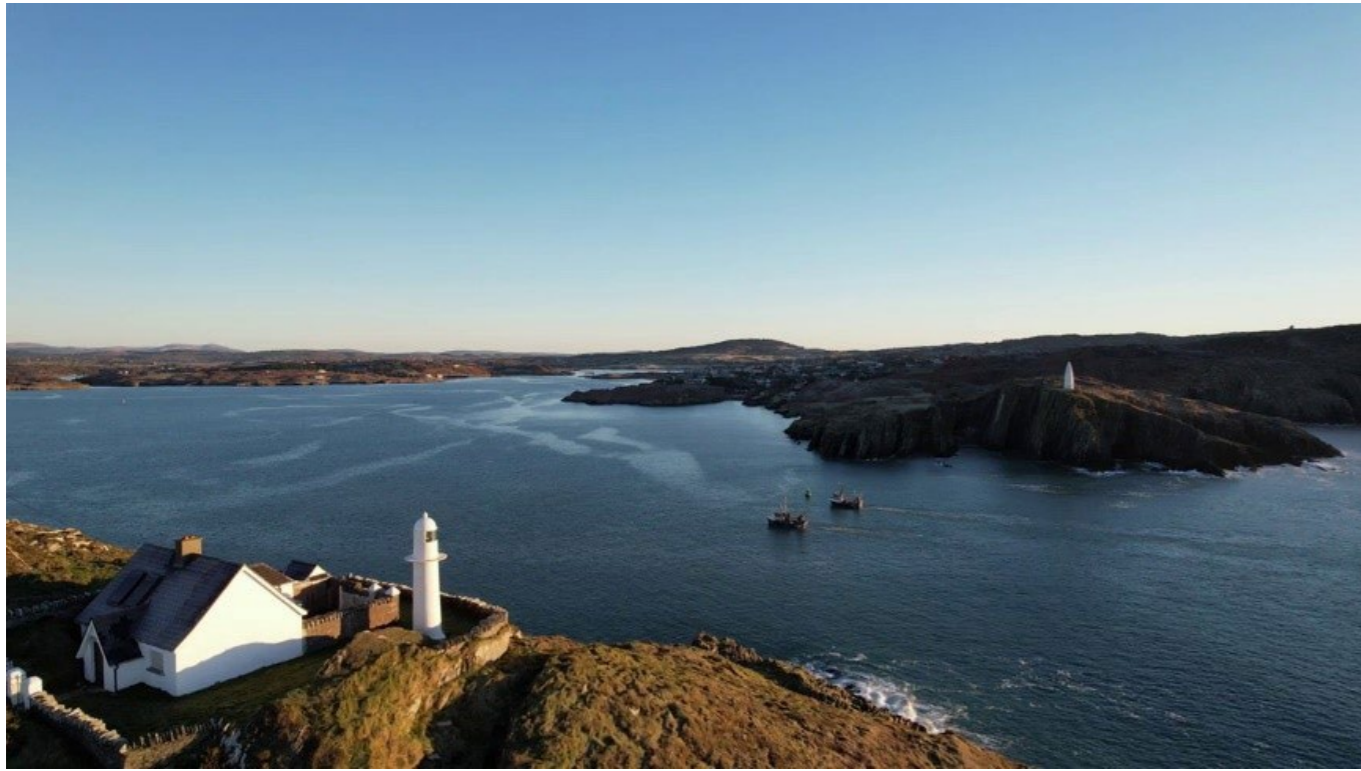
Refurbishment of Sherkin Lighthouse
