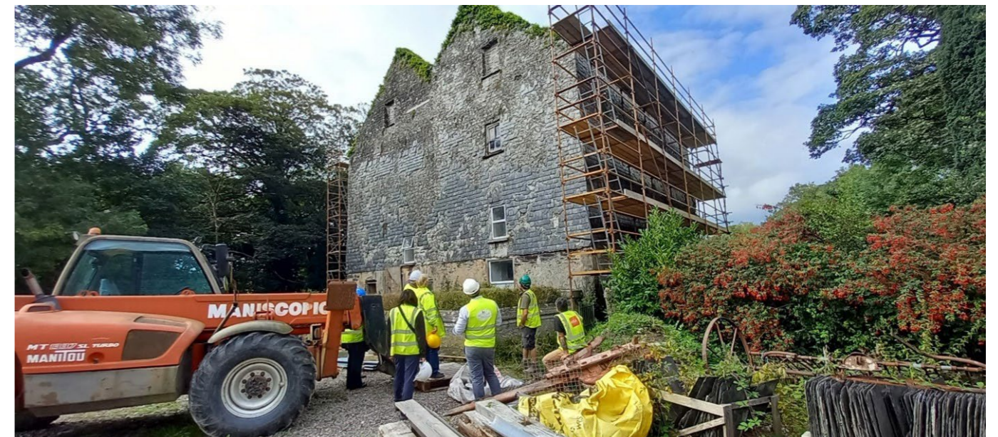
Castlevew Mills, near Clonakilty, received funding under the 2023 Community Monuments Fund
