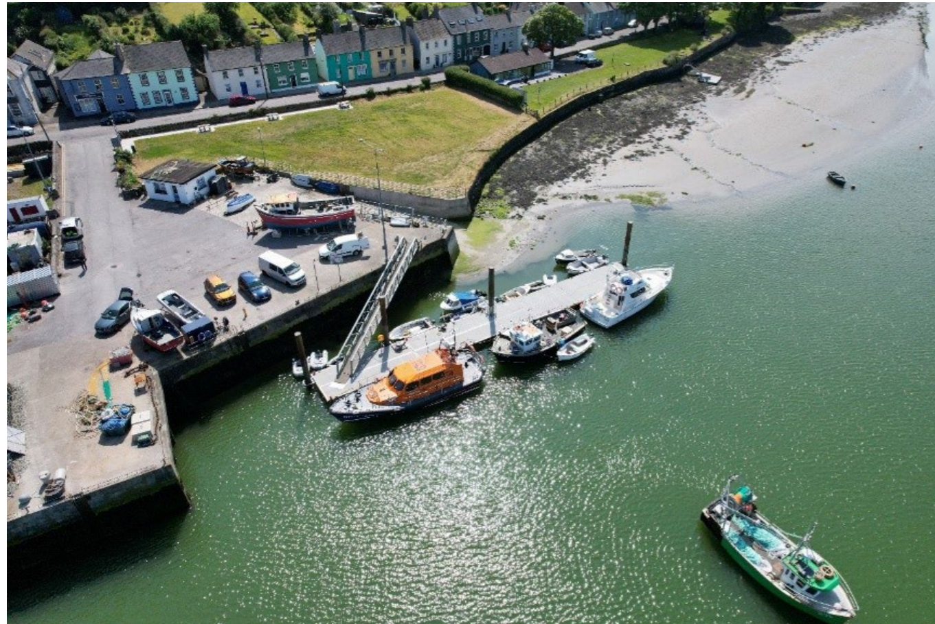
Courtmacsherry Dredging and Pontoon Replacement
