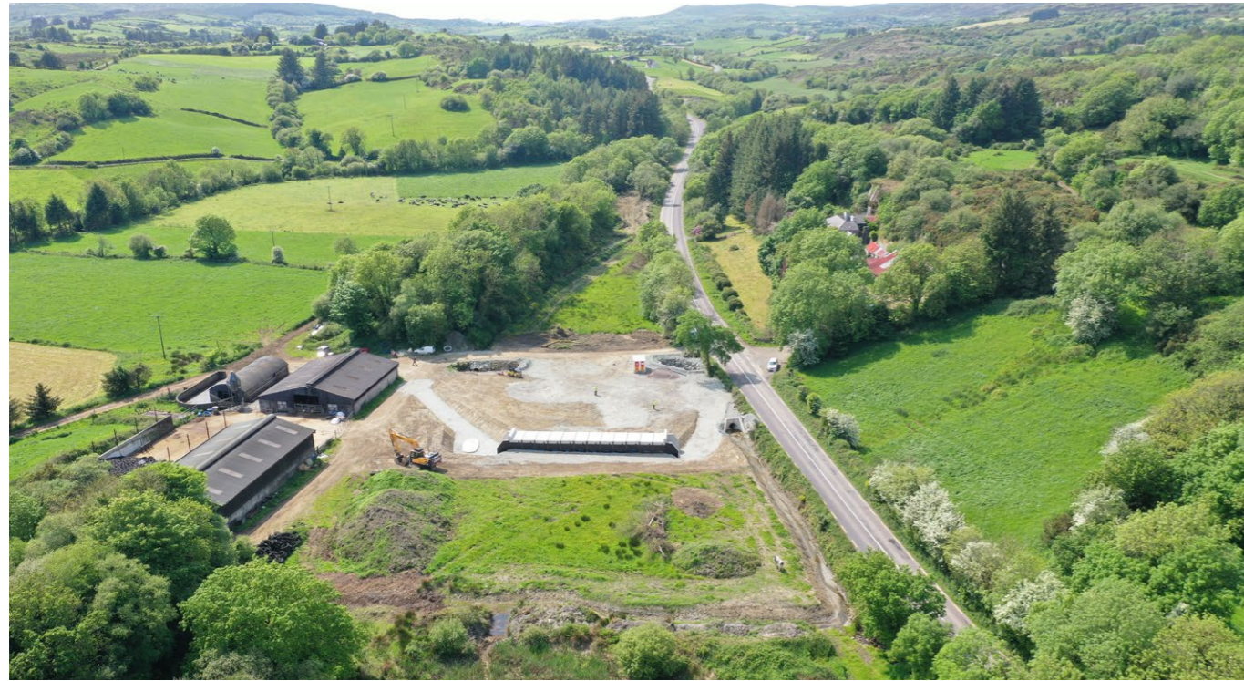
R586 realignment at Ilen Bridge
