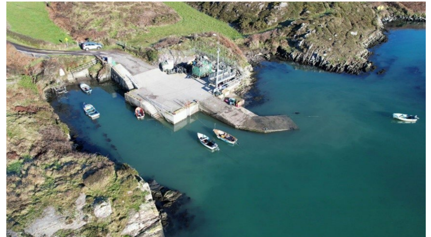
Turk Head Pier Improvement Works
