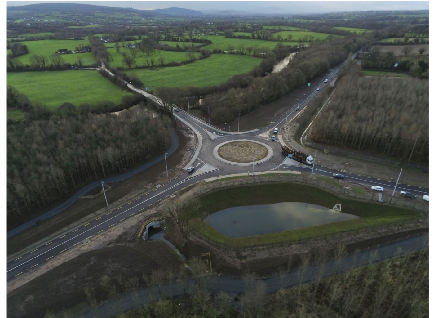
N72 Ballymaquirke Junction – Looking South-West
