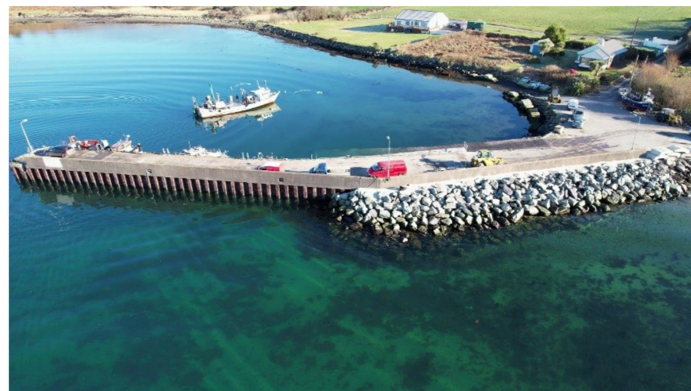
Laheratanvally Pier Remedial Works
