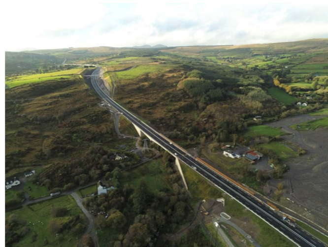
N22 Baile Bhuirne Macroom Road Development – Looking West toward Kerry with the Bohill River Bridge in the foreground.
