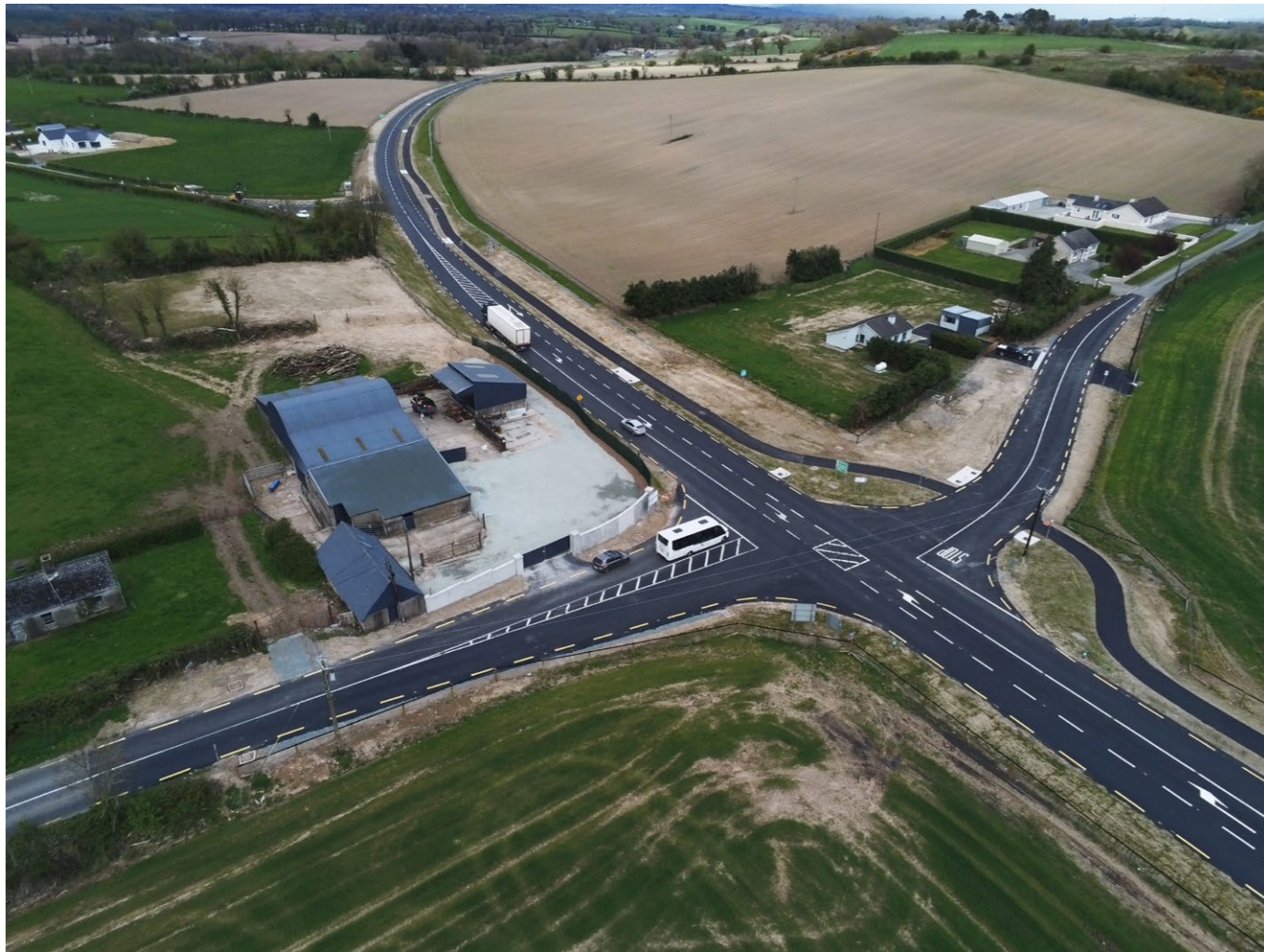
N73 Clogher Cross – Looking North-East
