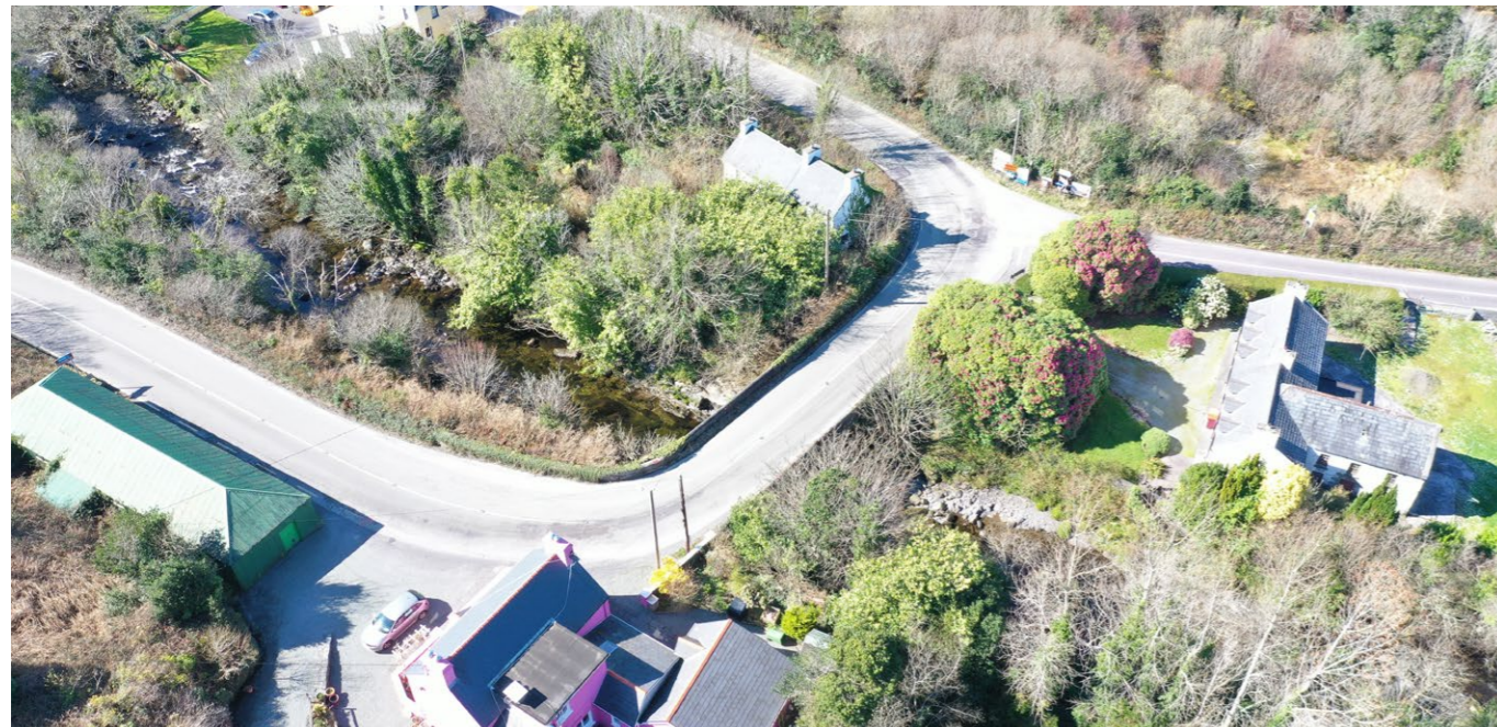
R572 realignment at Adrigole
