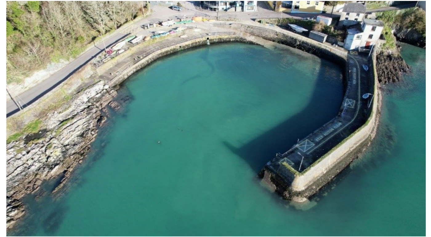
Glandore Pier Safety Improvement Work
