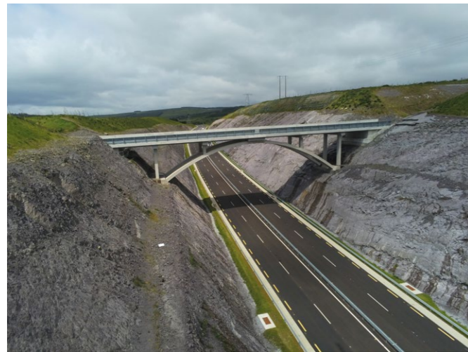
N22 Baile Bhuirne Macroom Road Development – 502C Concrete Arch Bridge at the top of Cut 1 on the Baile Bhuirne bypass section of the scheme.
