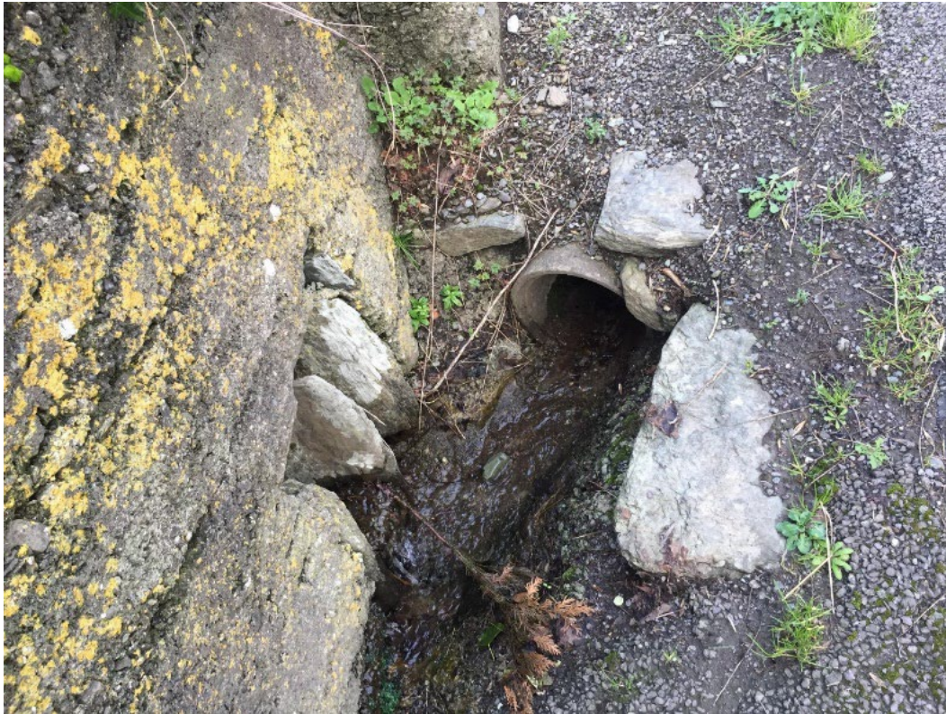
Figure 6. Drainage dyke hitting front boundary of site and running into underground drainage pipe.
