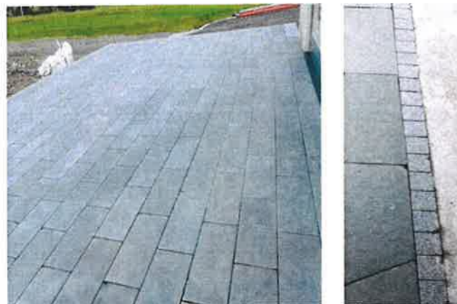
Limestons paving & edging
