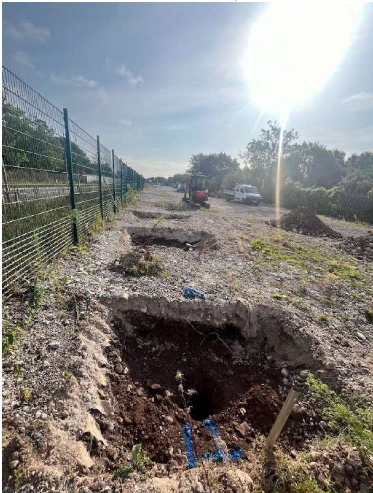
Excavated sub-surface test holes 1,2 and 3
