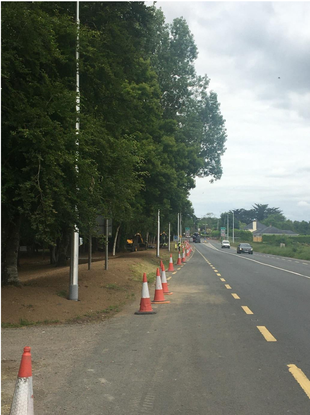
Typical scheme of passively safe columns on the N72 west of Mallow
