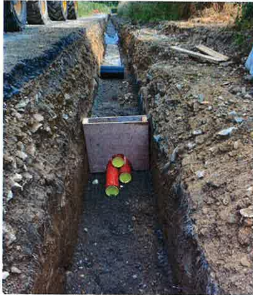
Figure 5-4 Typical 33KV Underground Duct Installation
